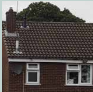
Glazed pantile roof
