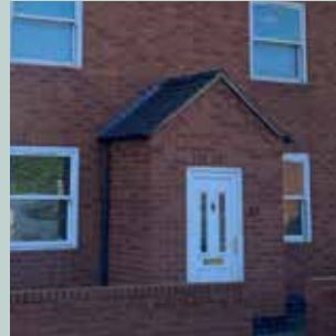
Gabled porch and detailing
