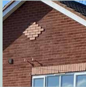
Brick detailing on wall
