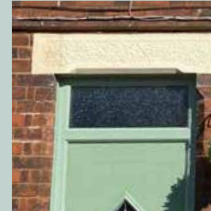
Lintel details on top of the door
