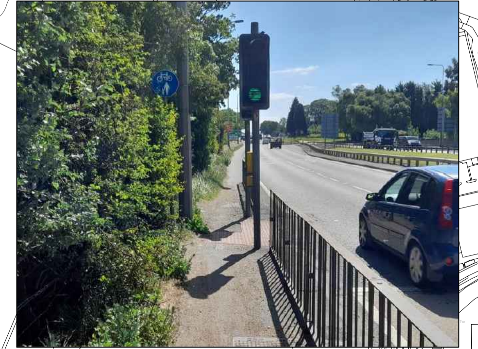
Existing Pinch Point on A5 Pavement / Cycleway at Birch Coppice Junction
