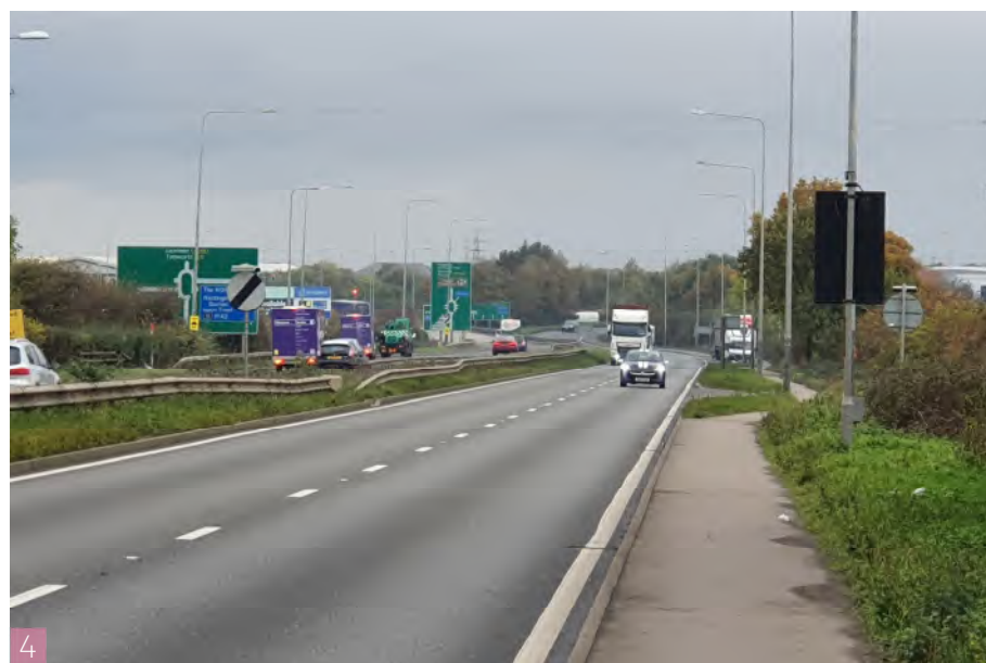
View of A5 dual carriageway facing west
