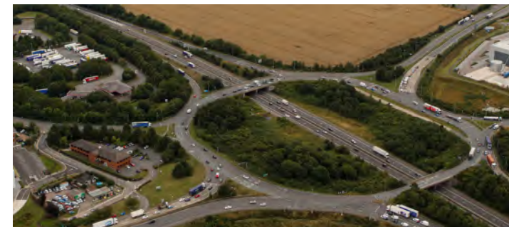
1. Junction 10 M42 Roundabout
