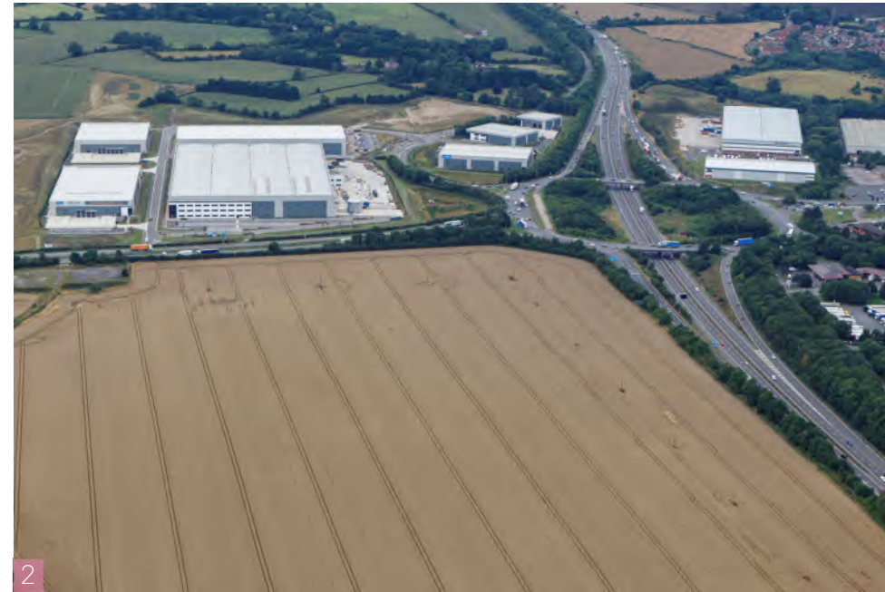
2 View looking south towards J10 M42
