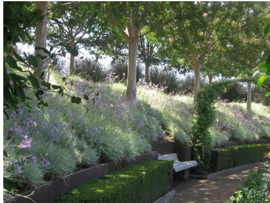
Landscaped retaining feature wall
