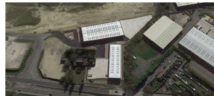
7. Hall End Hall Farm
