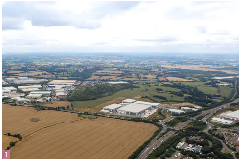
1 View looking south towards J10 M42
