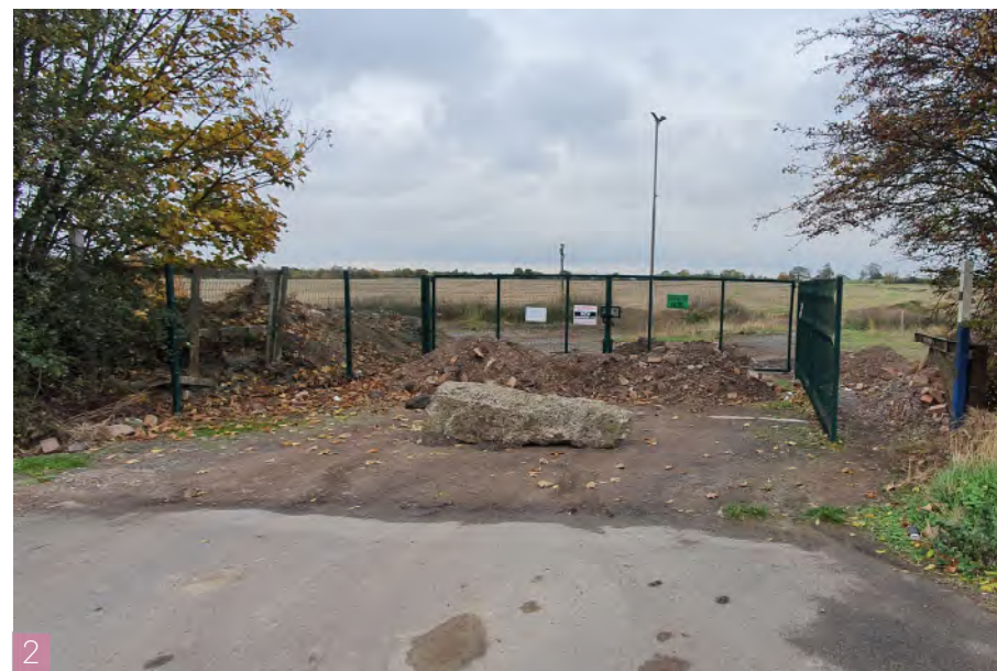
View south of existing site access
