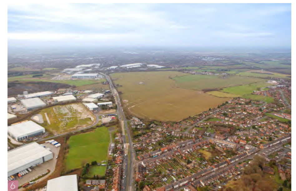
Aerial view of Site looking west from Dordon
