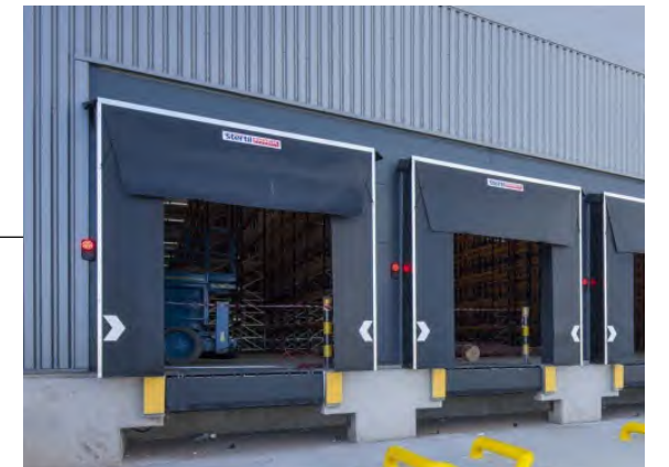
Dock Loading Doors
