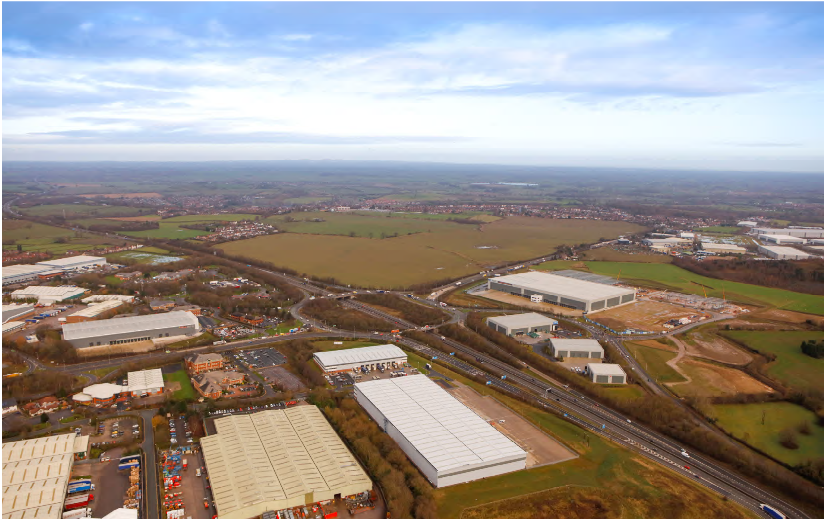
Fig. 1 – Aerial of Site Looking East from Junction 10 M42
