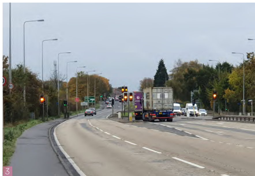
3 View eastwards to existing access junction for Birch Coppice Business Park
