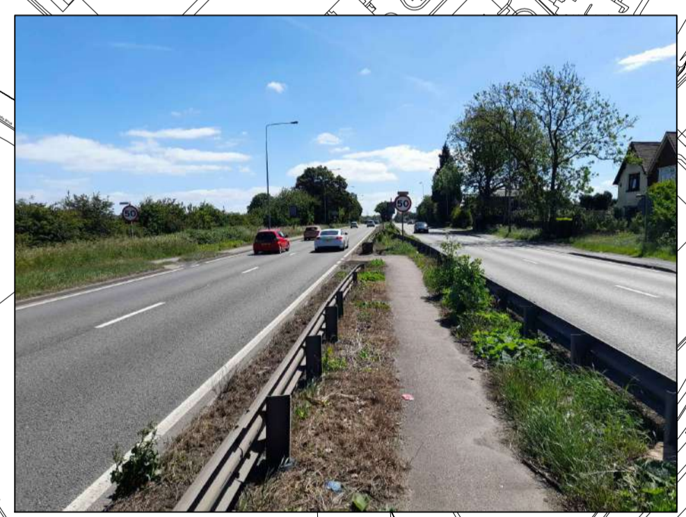
Existing Uncontrolled Staggered Pedestrian A5 Crossing - View East
