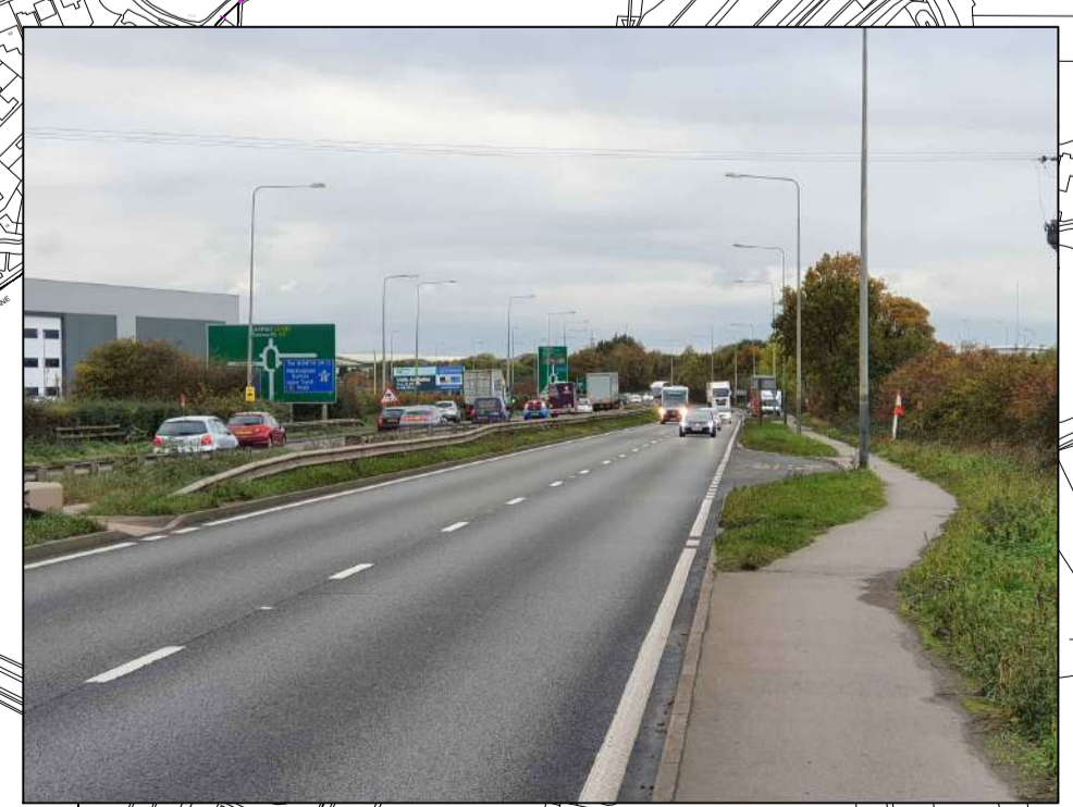
Existing Pinch Point on A5 Pavement / Cycleway at Bus Stop North of A5
