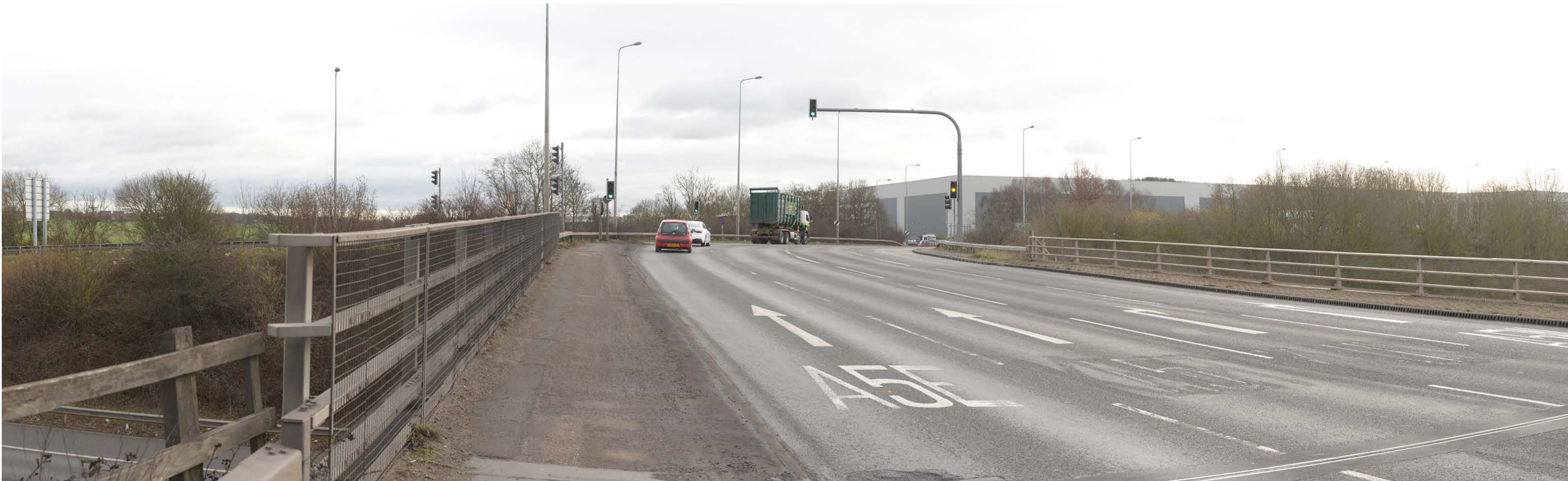
VIEWPOINT 13: LOOKING SOUTH-EAST TOWARDS THE SITE FROM THE FOOTPATH AT JUNCTION 10.
