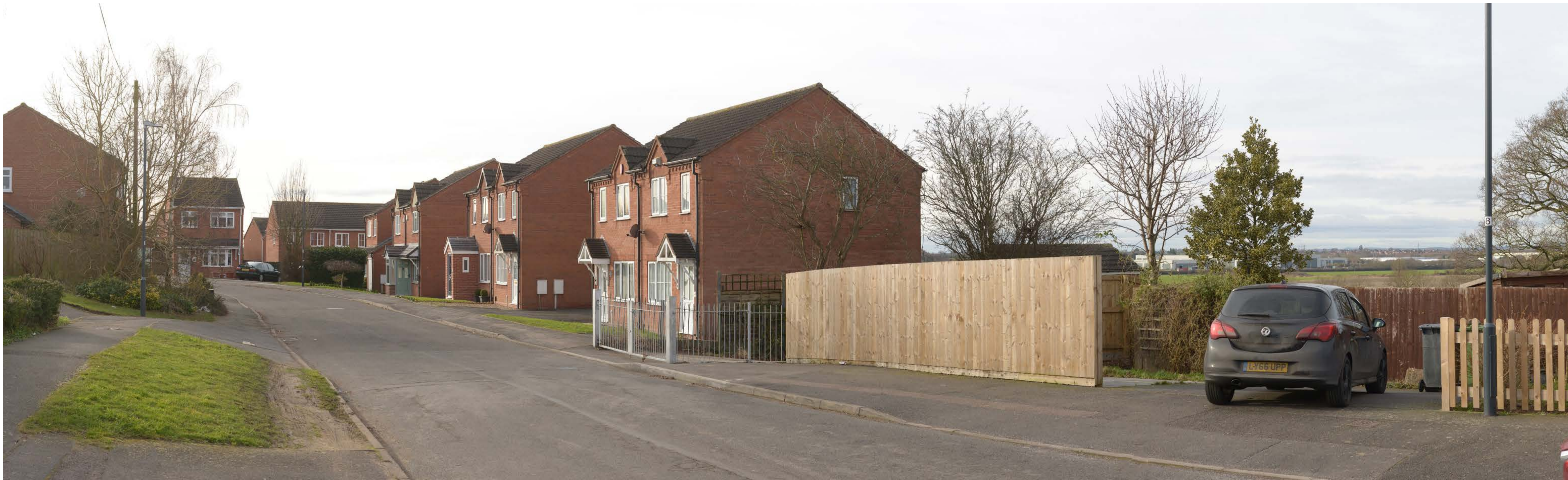
VIEWPOINT 19: LOOKING SOUTH TOWARDS THE SITE FROM OFF BIRCHWOOD AVENUE AT ENTRANCE TO TOMLINSON CONSTRUCTION SITE.
