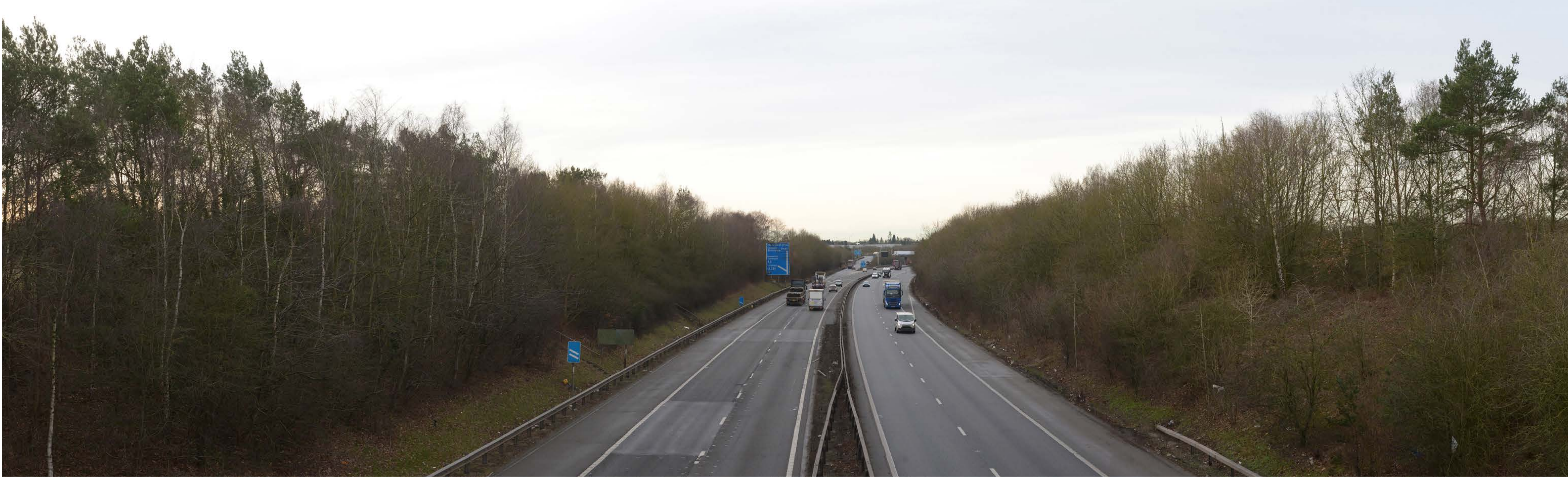
VIEWPOINT 16: LOOKING SOUTH ALONG THE M42 TOWARDS JUNCTION 10 FROM THE BRIDGE AT BIRCHMOOR.
