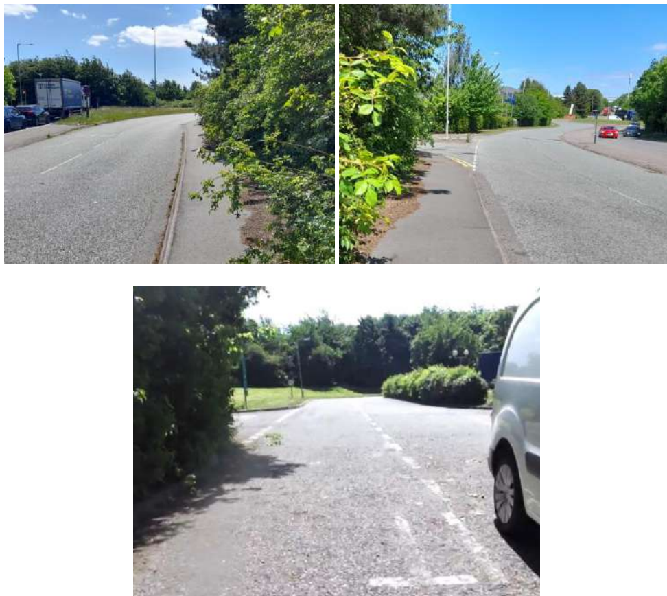
Figure 7 – Relay Drive/ Tamworth Services
