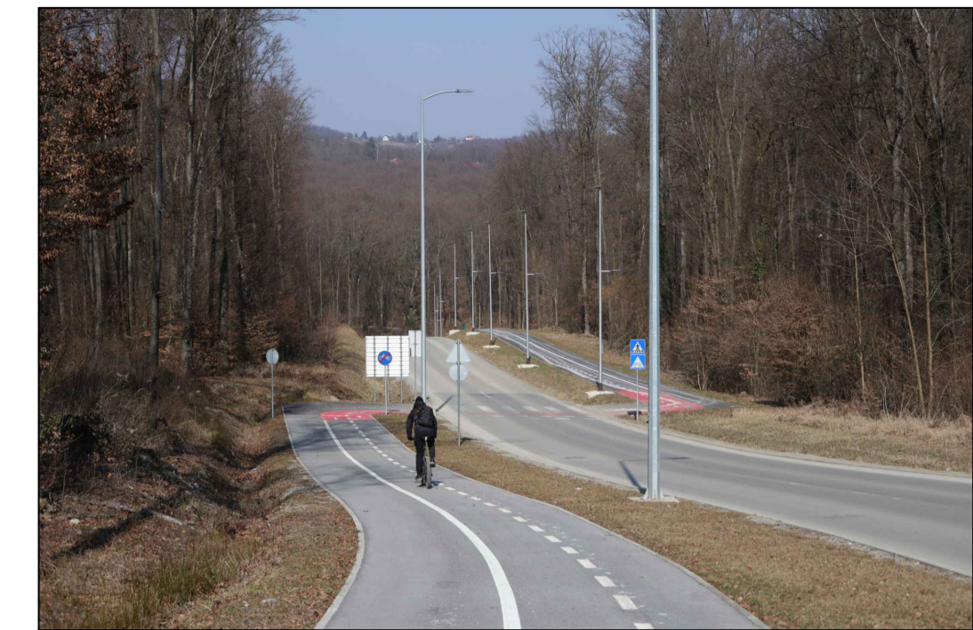
Dual 3m wide tarmacked footway/cycleways for the new pedestrian/cycle routes
