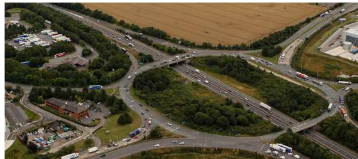
1 Junction 10 M42 Roundabout
