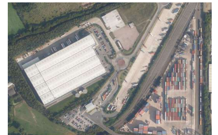
4 Birmingham Intermodal Freight Terminal (BIFT)
