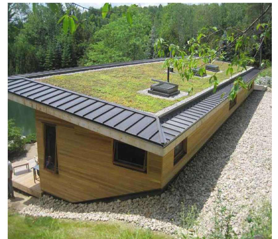
Example of Green Roof
