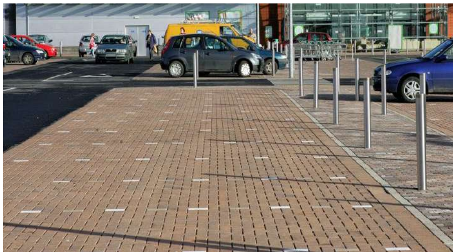
Car park areas constructed with macadam and permeable blockwork
