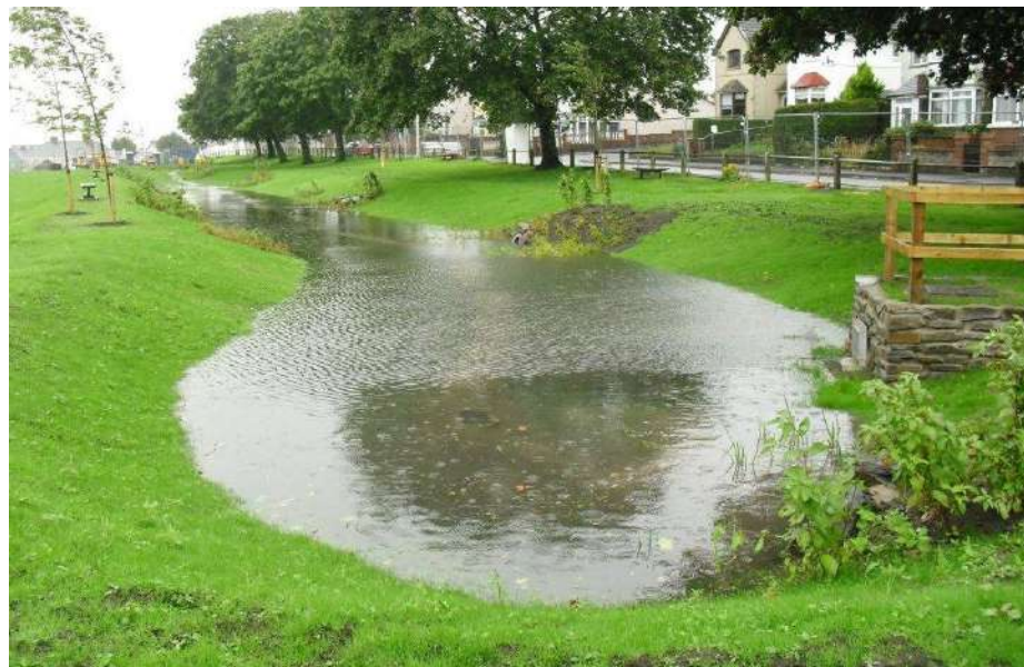
Sustainable Drainage Systems
