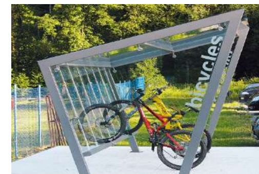
Covered cycle storage
