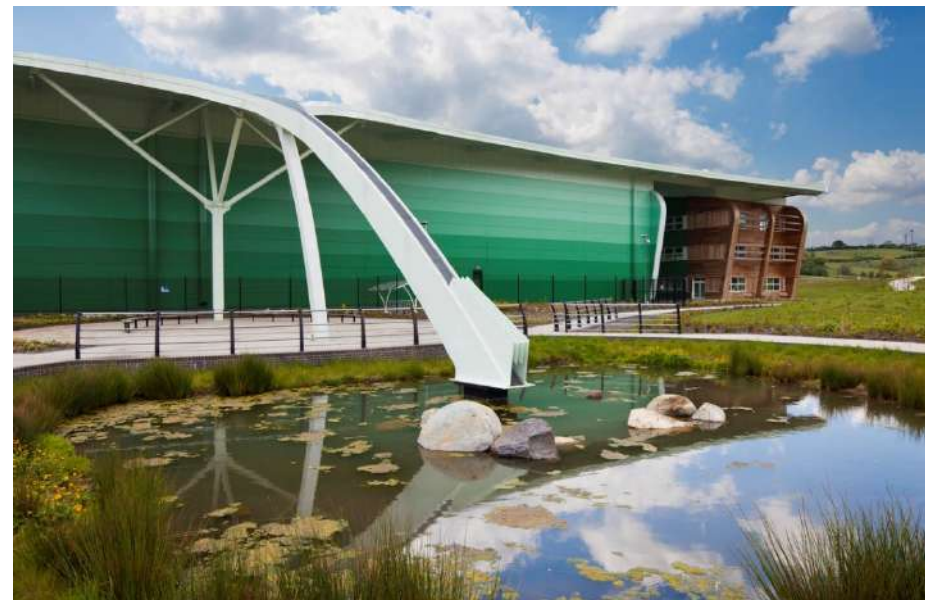
Dynamic roof controls runoff into attenuation pond
