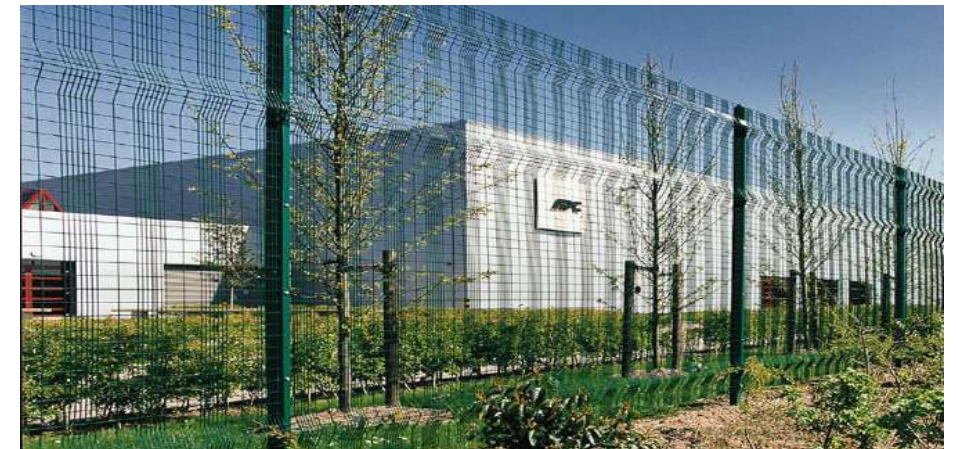
2.4m high palisade fencing
