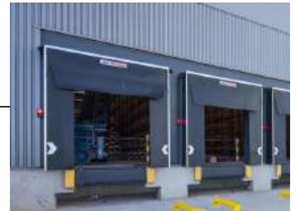
Dock Loading Doors
