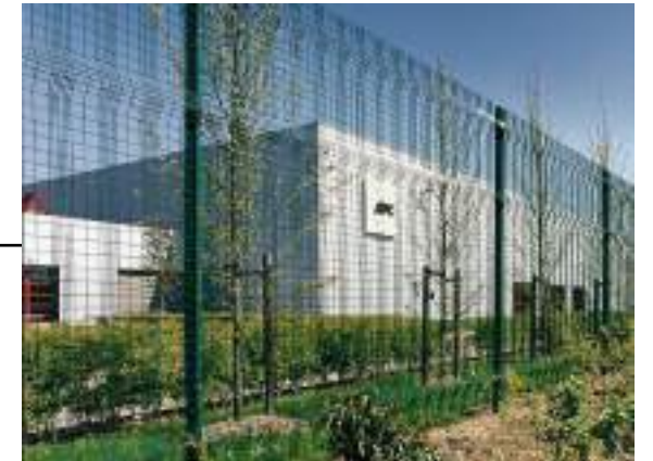
Fencing and Security
