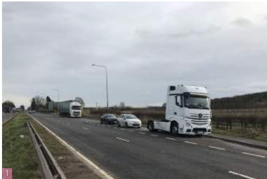
1 View looking east towards layby on westbound A5
