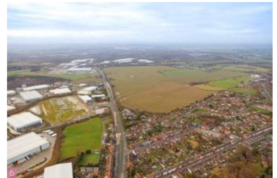
6 Aerial view of Site looking west from Dordon
