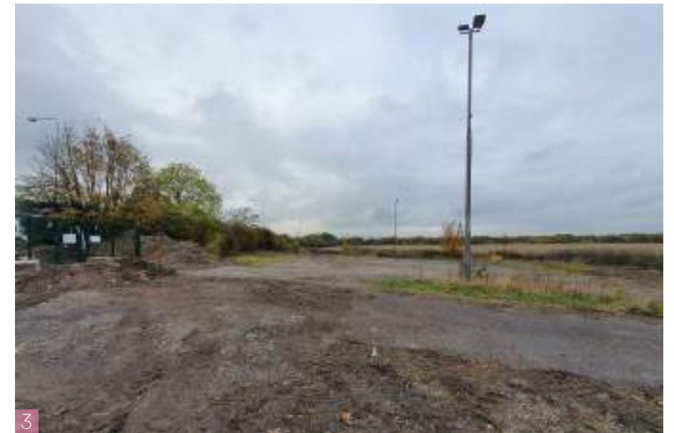
3 Existing hardstanding in the south of the Site looking west
