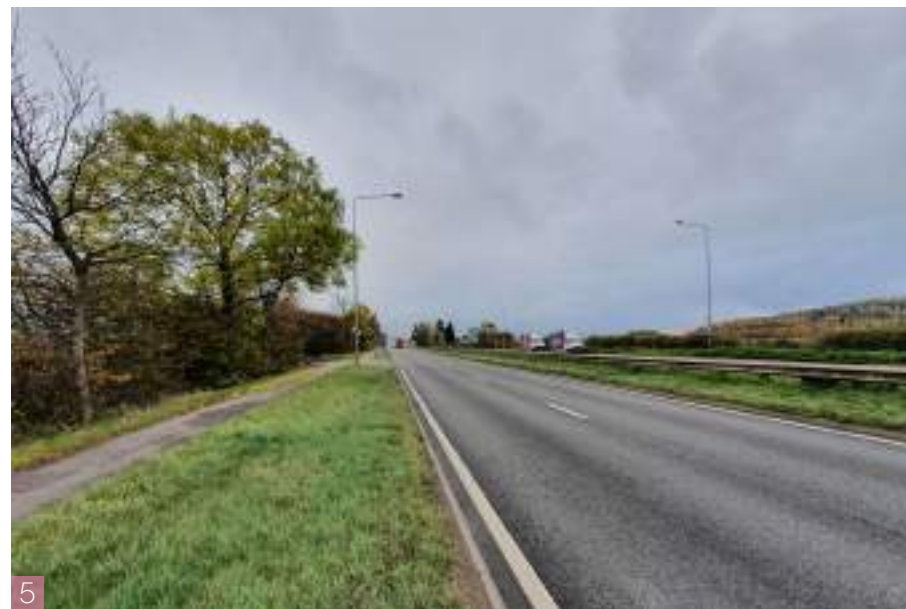
5 View of A5 dual carriageway facing east
