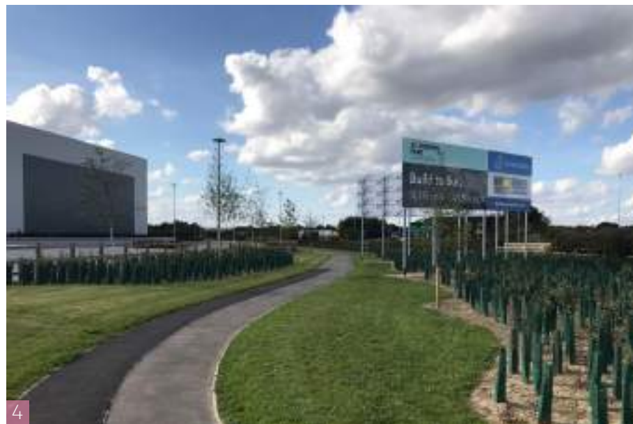
4 View west of landscaping along A5 corridor at St Modwen Park Tamworth
