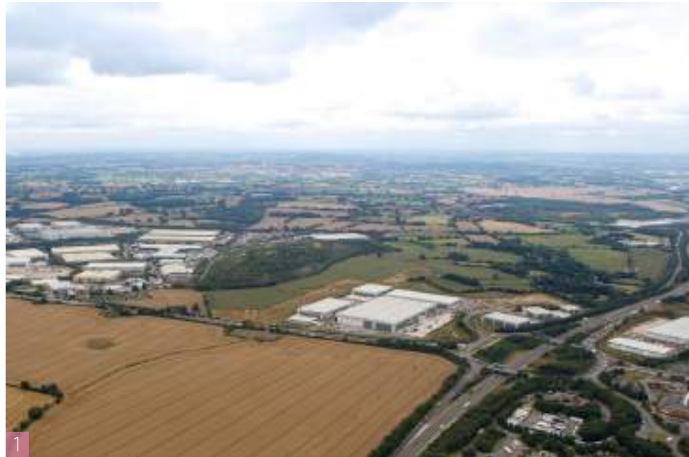
1 View looking south towards J10 M42
