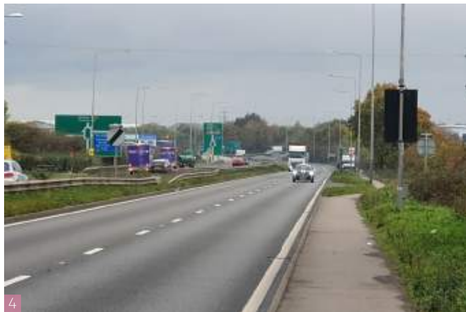
4 View of A5 dual carriageway facing west
