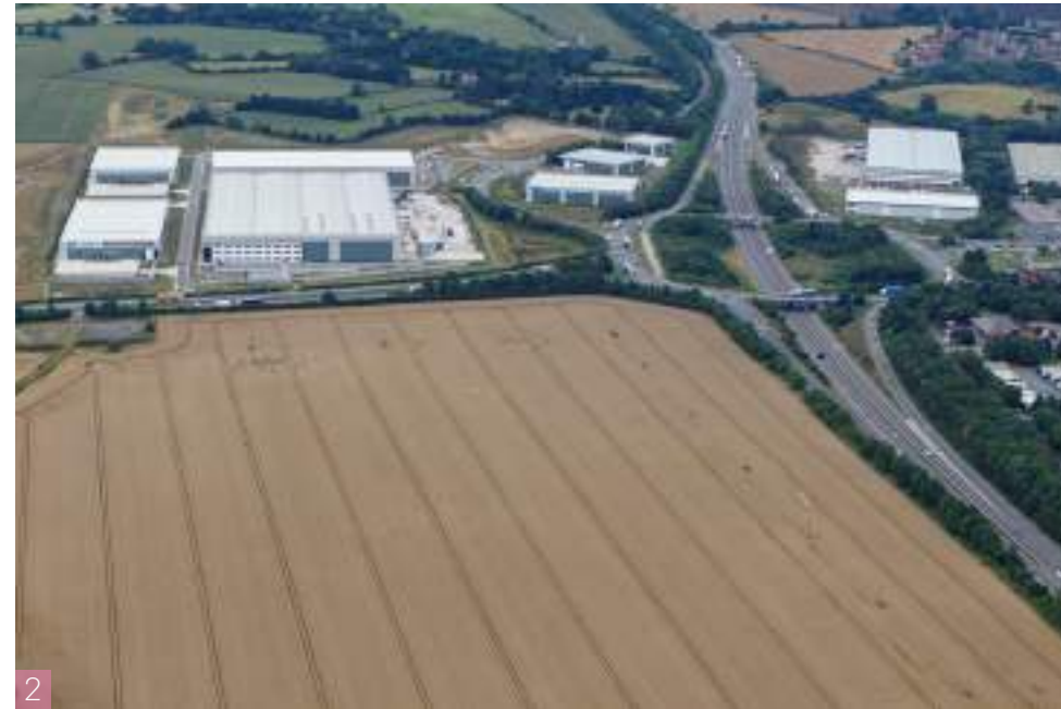
2 View looking south towards J10 M42
