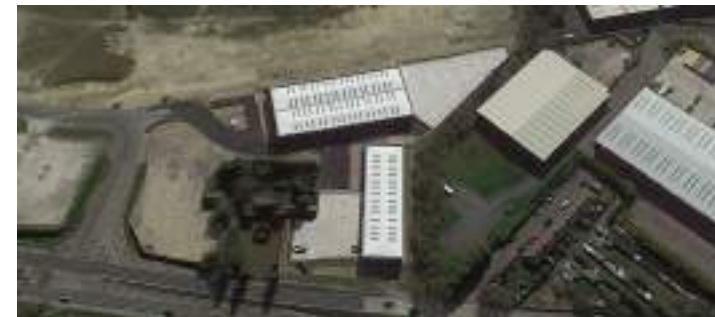
7. Hall End Hall Farm
