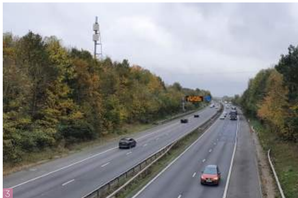
3 View south from Green Lane bridge over M42
