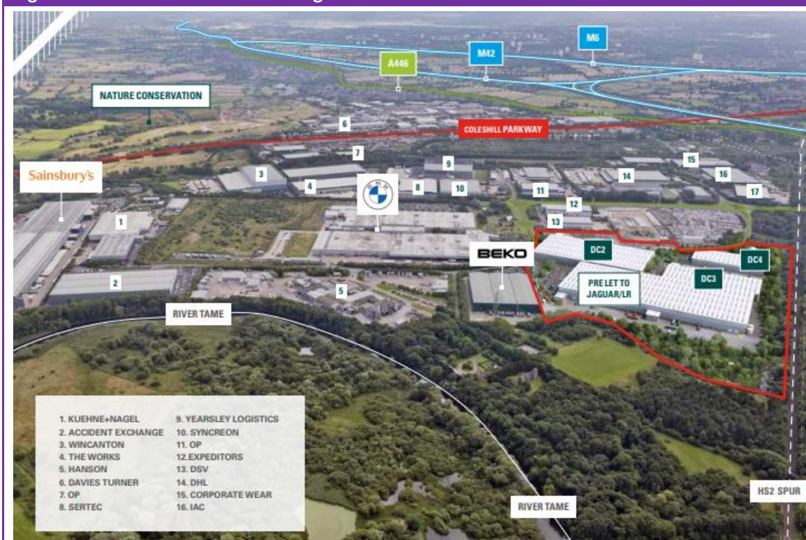
Figure 2.8: Hams Hall Manufacturing and Distribution Park
