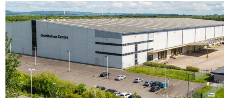
W248 Building 1000, Western Approach Bristol – Wincanton 248,000 sq ft
