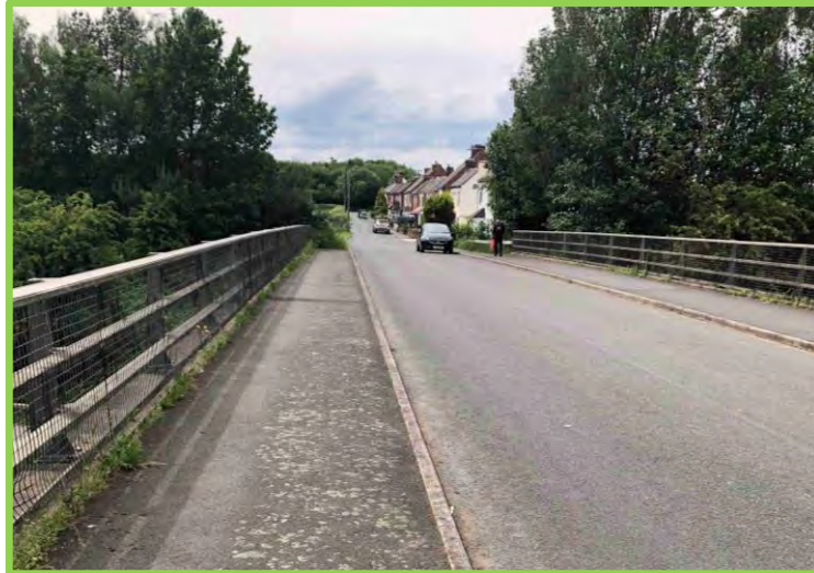
footways on Green Lane
