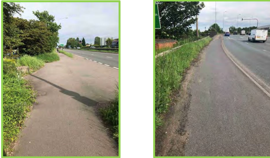
Existing footways at site frontage on A5 (left) and at northern edge of M42 Junction 10 (right)
