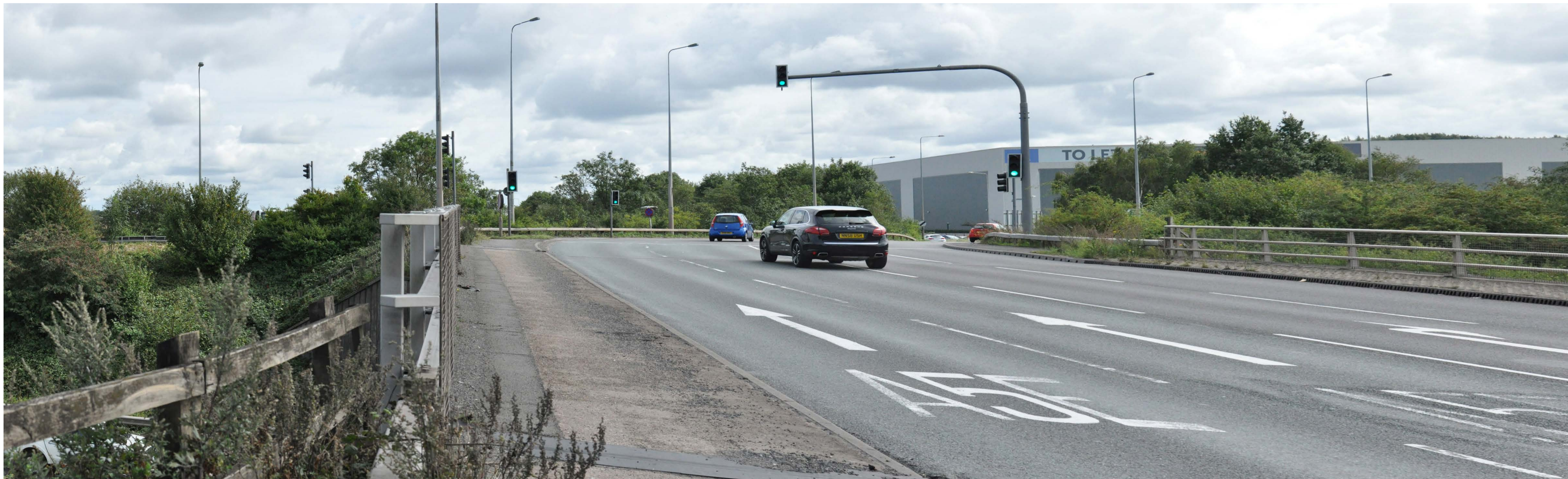
VIEWPOINT: 14 LOOKING SOUTH-EAST TOWARDS THE SITE FROM THE FOOTPATH AT JUNCTION 10.
