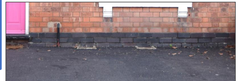
Raised ground levels at 2-12 Vicarage Lane
