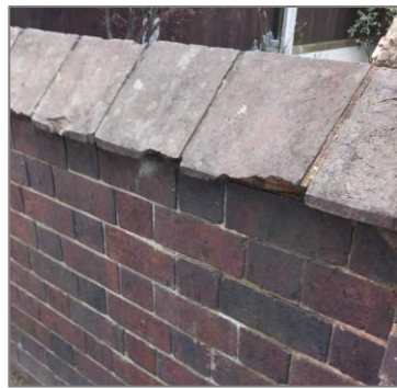
An old example of a blue brick wall with matching coping.
