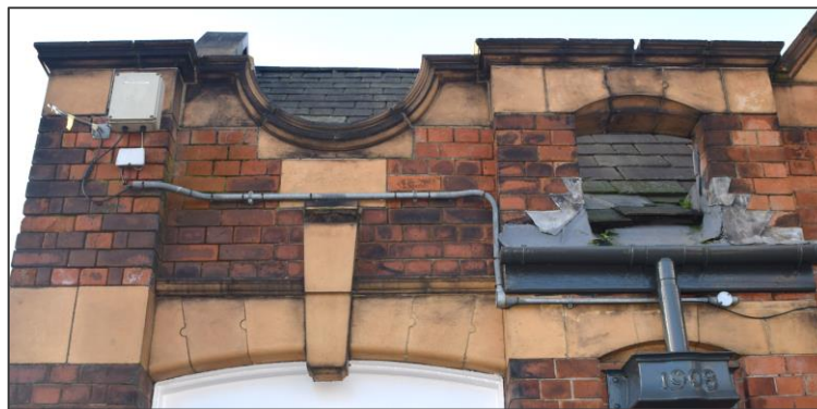
Faience (glazed terracotta) used in the Train Station as a decorative, but affordable material.
