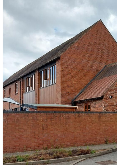
This barn range at the Courtyard is built of English bond brickwork, giving its walls a very solid appearance. The later single storey extension and boundary walls are of different brick laid in different bonds, but the use of red bricks and red clay roofs unites the new and old.
