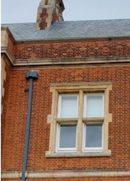
Detail of Caldecote Hall. The smooth stone dressings and Flemish bond brickwork form a visually pleasing contrast.
