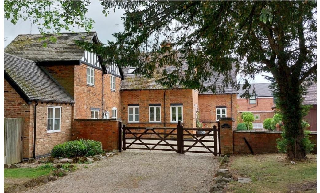
The Mews, Caldecote Hall
