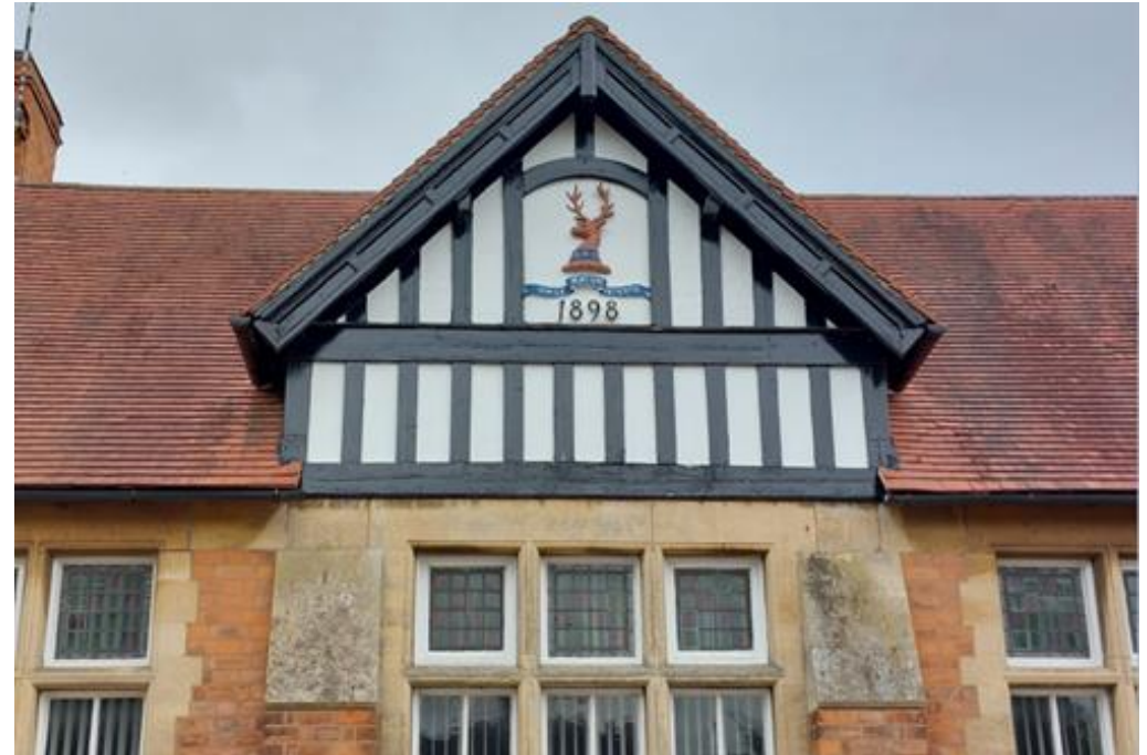
Figure 3.3: Village hall gable
