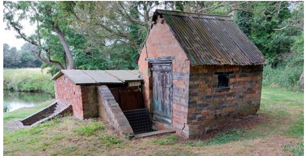
Figure A.4: The powerhouse in the grounds of Caldecote Hall
