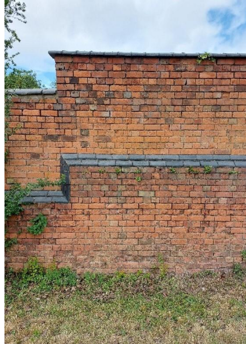
The brick garden wall to the Hall kitchen garden is constructed in English bond (alternating beds of headers and stretchers). By making the wall thinner halfway up its height, it could be built without the need for buttresses or piers. The blue clay copings to the lower and upper sections of wall help to keep the brickwork dry.
