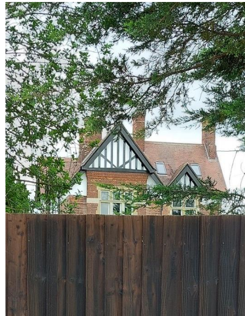
The steep gables and multiple chimneystacks of the Grange, built as the Rectory and second only to the Hall in status when it was built.
