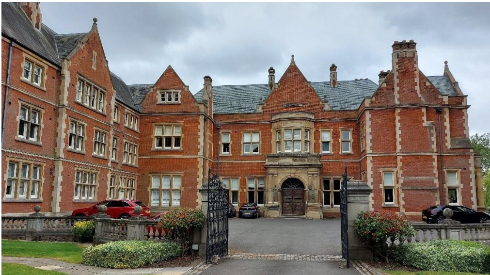
Figure A.1: Caldecote Hall principal entrance
