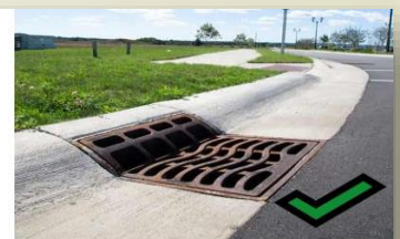
combination 'well' and kerb drain, set into concrete roadside edging
