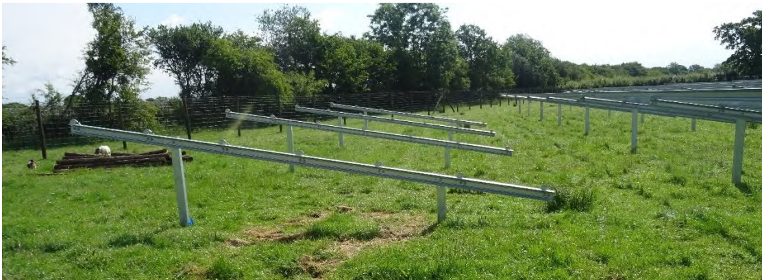
Piles Installed (this is at Bentham Farm, Purton, Summer 2015)
