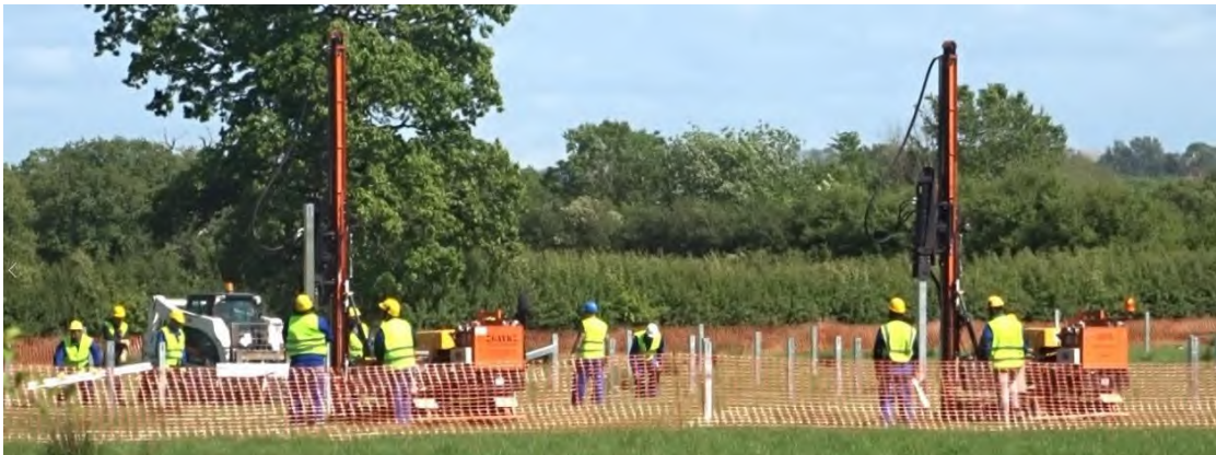
Piles Being Installed
