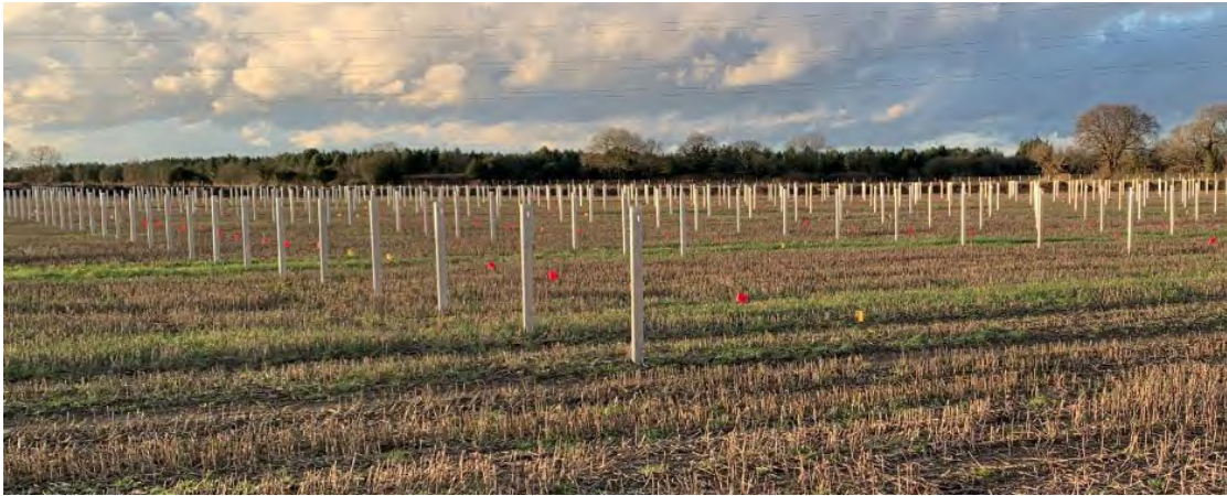
Piles Being Installed (this is at Tilt Farm, Retford, in January 2023)
