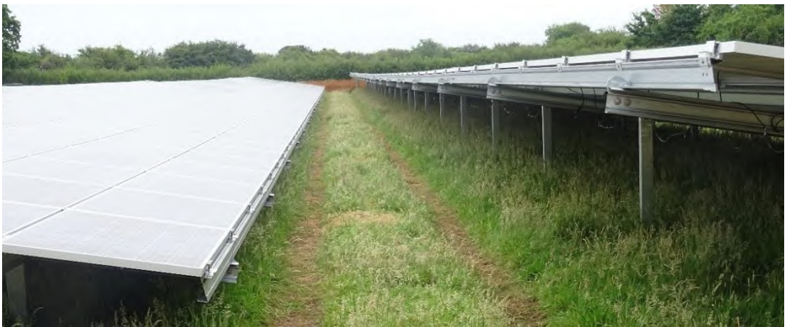
After Panels Bolted-On
