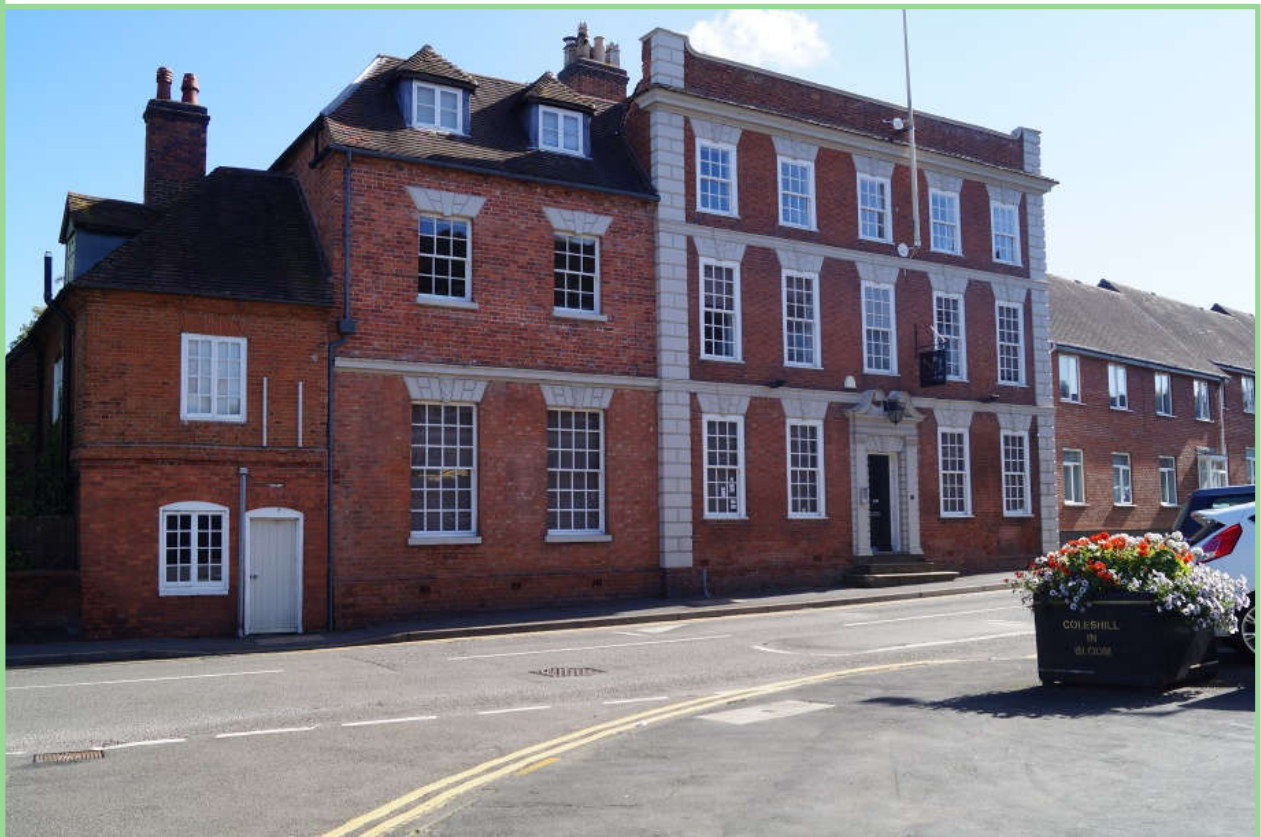
Offices and Accommodation in Coleshill High Street North
