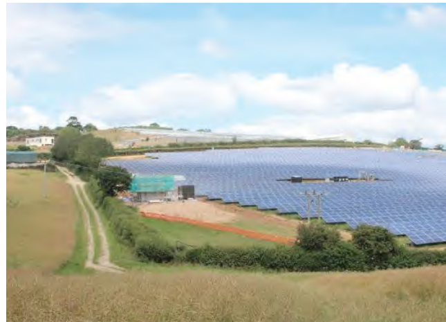
Figure 17 The 5MW Howton solar farm in Cornwall. Image courtesy of Lightsource Limited.
