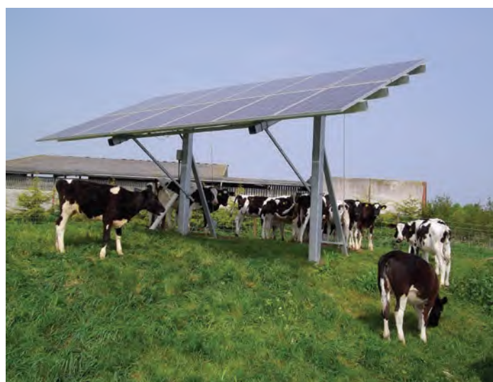
Figure 4 Sheep and cattle grazing under solar panel arrays. Support structures, and the height of panels, would need to be substantial in order to allow cattle grazing and would not ordinarily be recommended. Images courtesy of Steve Edmunds, Mole Valley Renewables.
