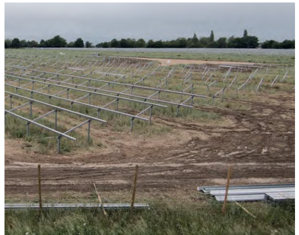
View from Turpin's Trail during Terrier's Farm construction
