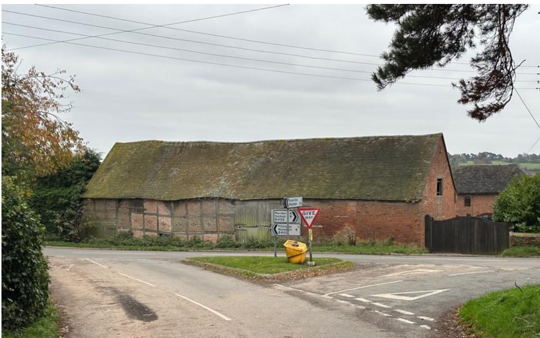
Figure 4 Grade II listed early 17 th century threshing barn at Park House Farm, looking east.
