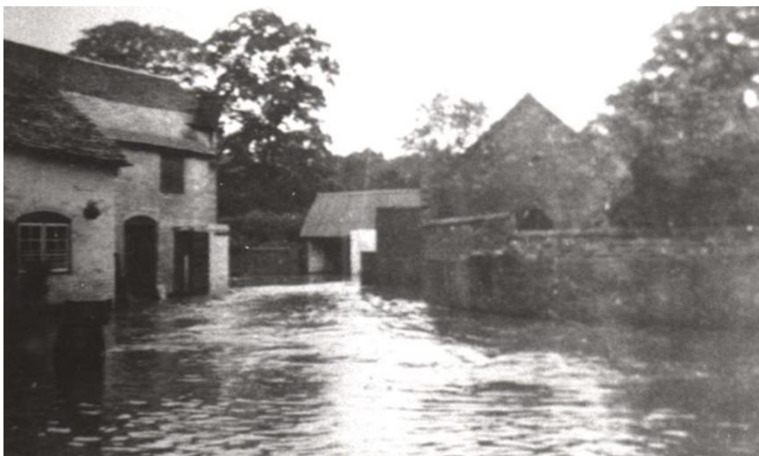
Figure 20 The Bell public house in Fillongley in the early 1900s flooded by waters from the Bourne Brook.
