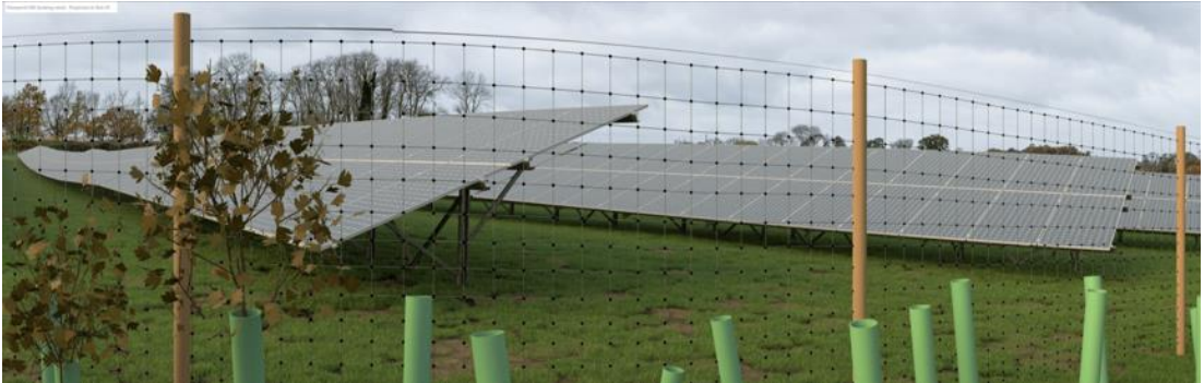
Figure 34 Proposed view south from the historic footpath within the site. Source: Andy Maw Design.
