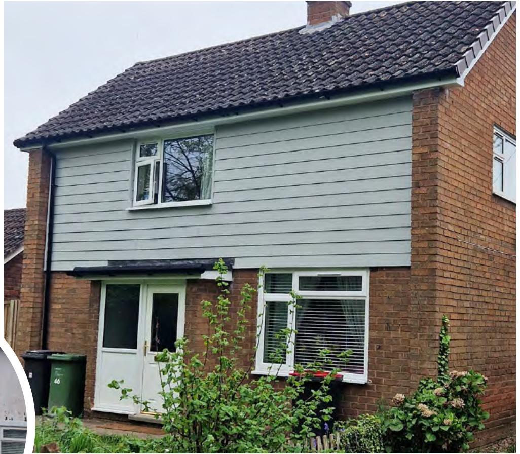
After photograph of property in Coleshill following external cladding, replacement fascia boards and guttering.
