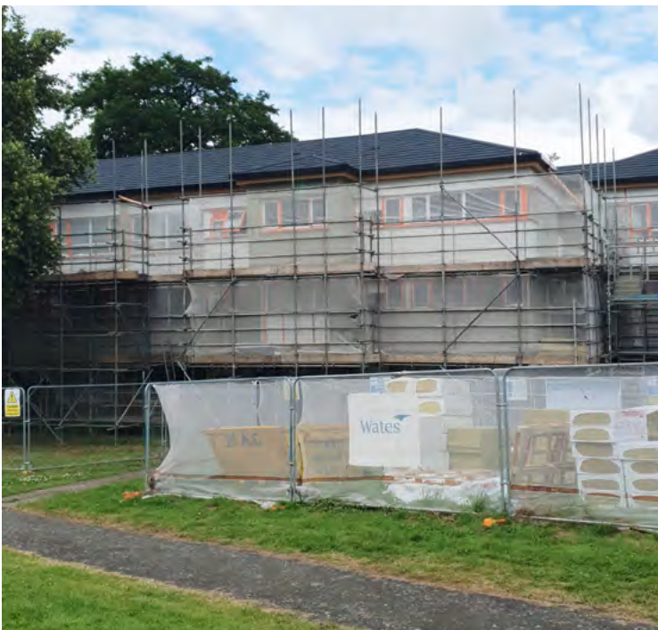
Ongoing improvement work at Abbey Green Court, Polesworth.
