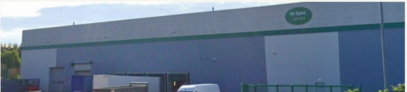
Parapet (Hidden) Roof
