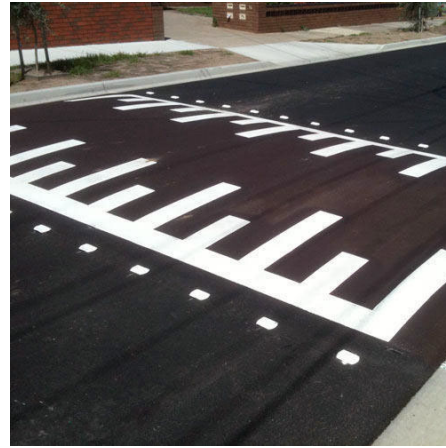
Reflective Road Marking
