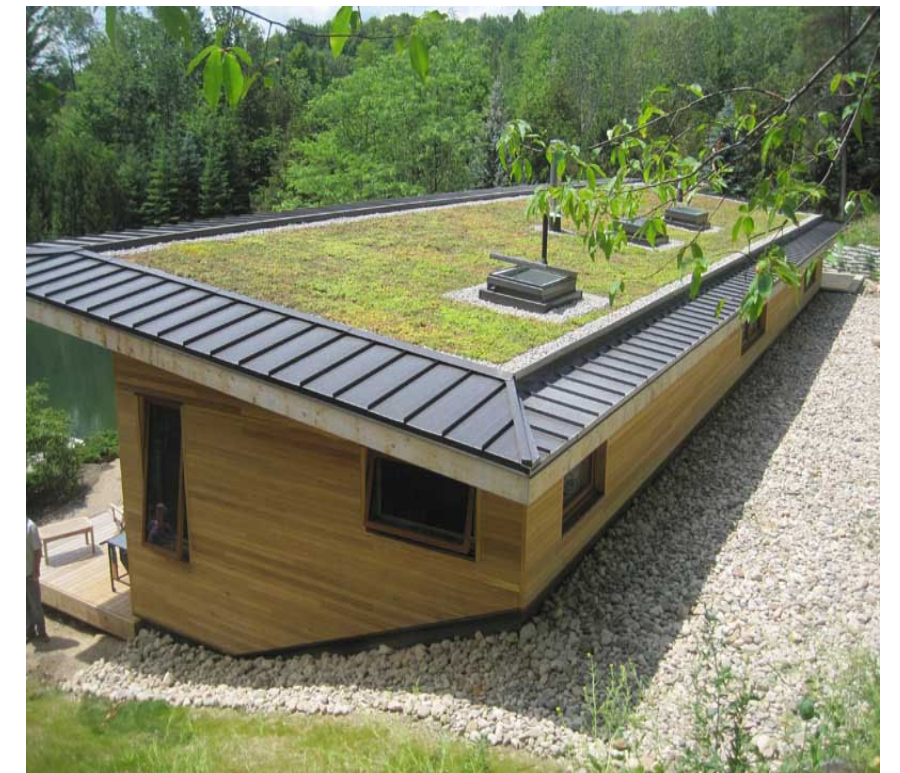
Example of Green Roof
