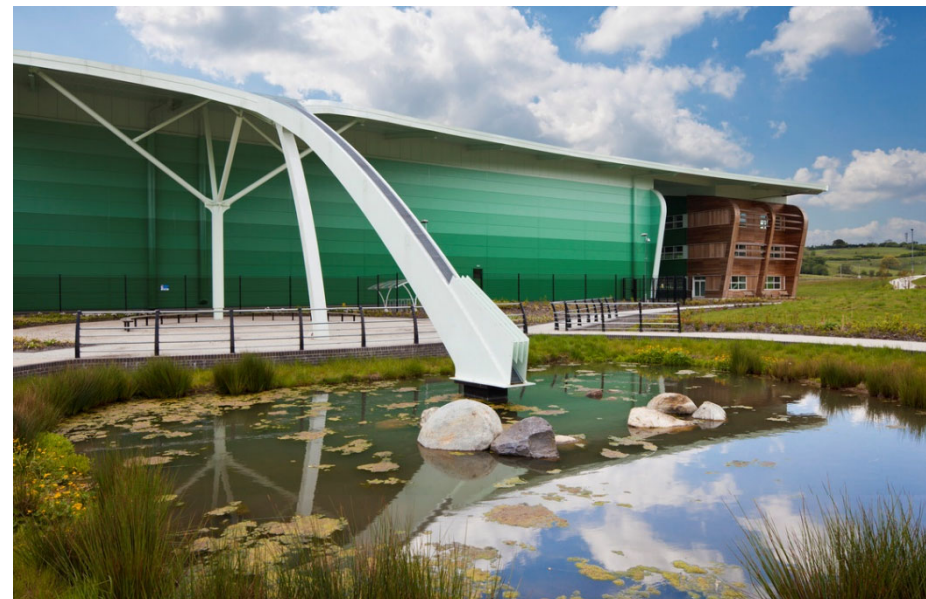
Dynamic roof controls runoff into attenuation pond
