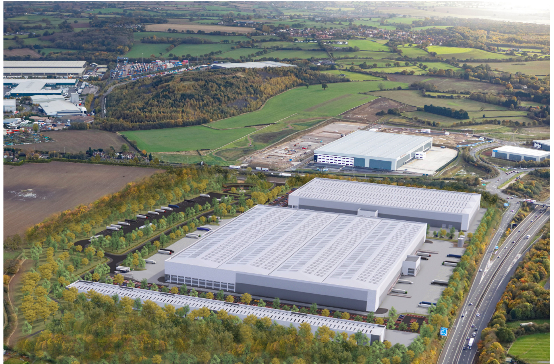
Proposed development to include industrial warehouses, a secure overnight lorry parking facility, substantial area of green infrastructure, enhance the existing interface and access point, provide new pedestrian and cycle routes, incorporate sustainable measures.
