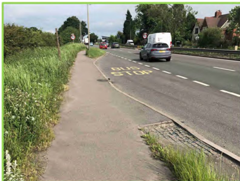
Existing bus stop facilities at A5 eastbound
