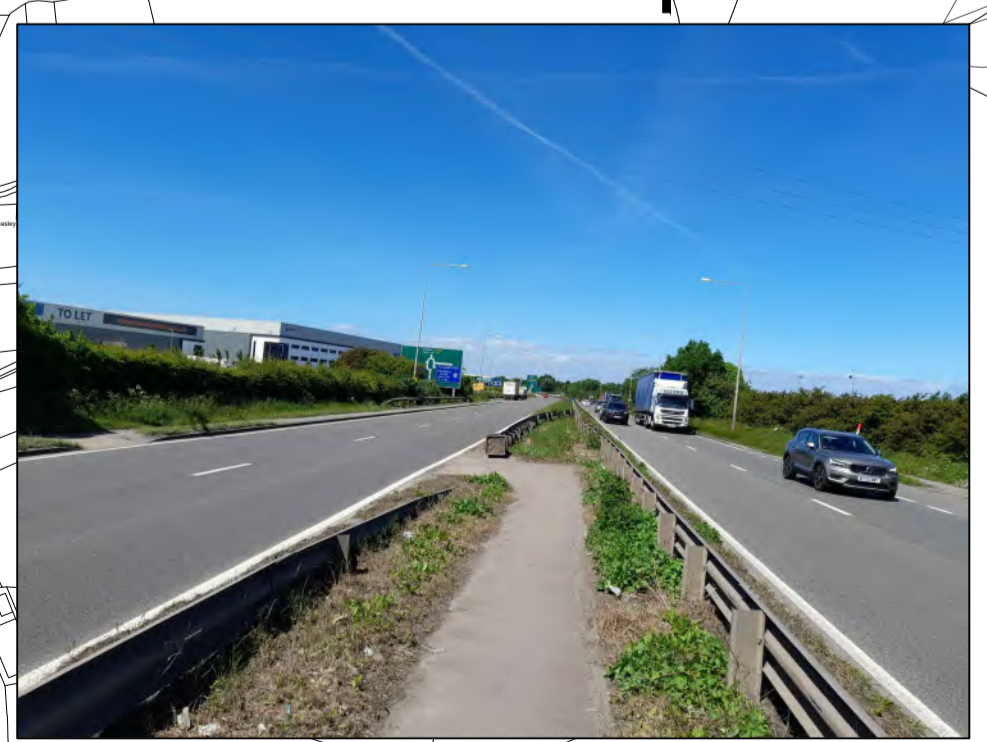
Existing Uncontrolled Staggered Pedestrian A5 Crossing - View West
