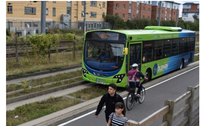
A guided busway with dedicated pedestrian and cycle paths provides fast and direct links to connect new and existing neighbourhoods with employment and services in Cambridgeshire .
