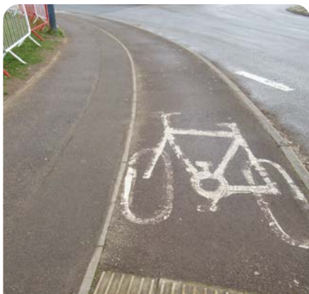
Kerb segregated cycle track, Warwick
