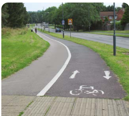
Raised white line segregated cycle track with tactile surfacing, Leamington
