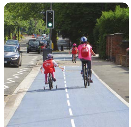
Kerb segregated two-way cycle track alongside road, Birmingham
