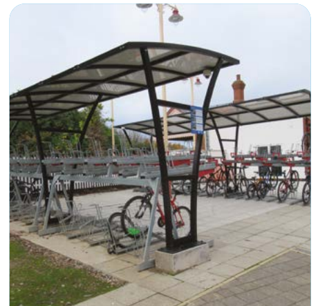
Two-tier covered cycle parking, Stratford
