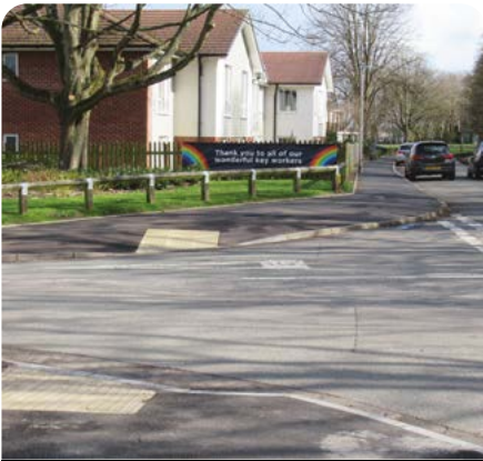
Resurfaced footway with tactile paving, Atherstone
