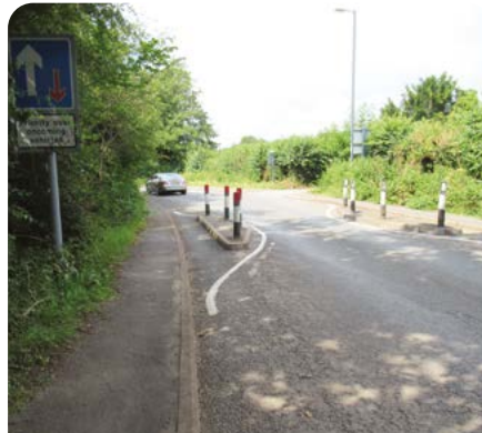
Horizontal traffic calming (give-way with cycle bypasses), Baginton
