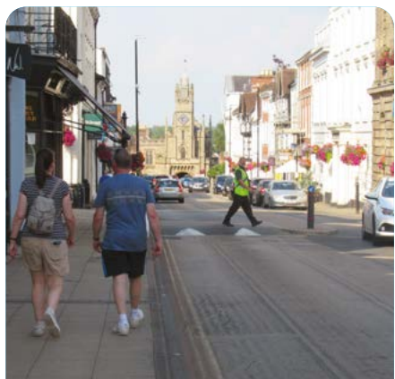
Raised crossing point, Warwick
