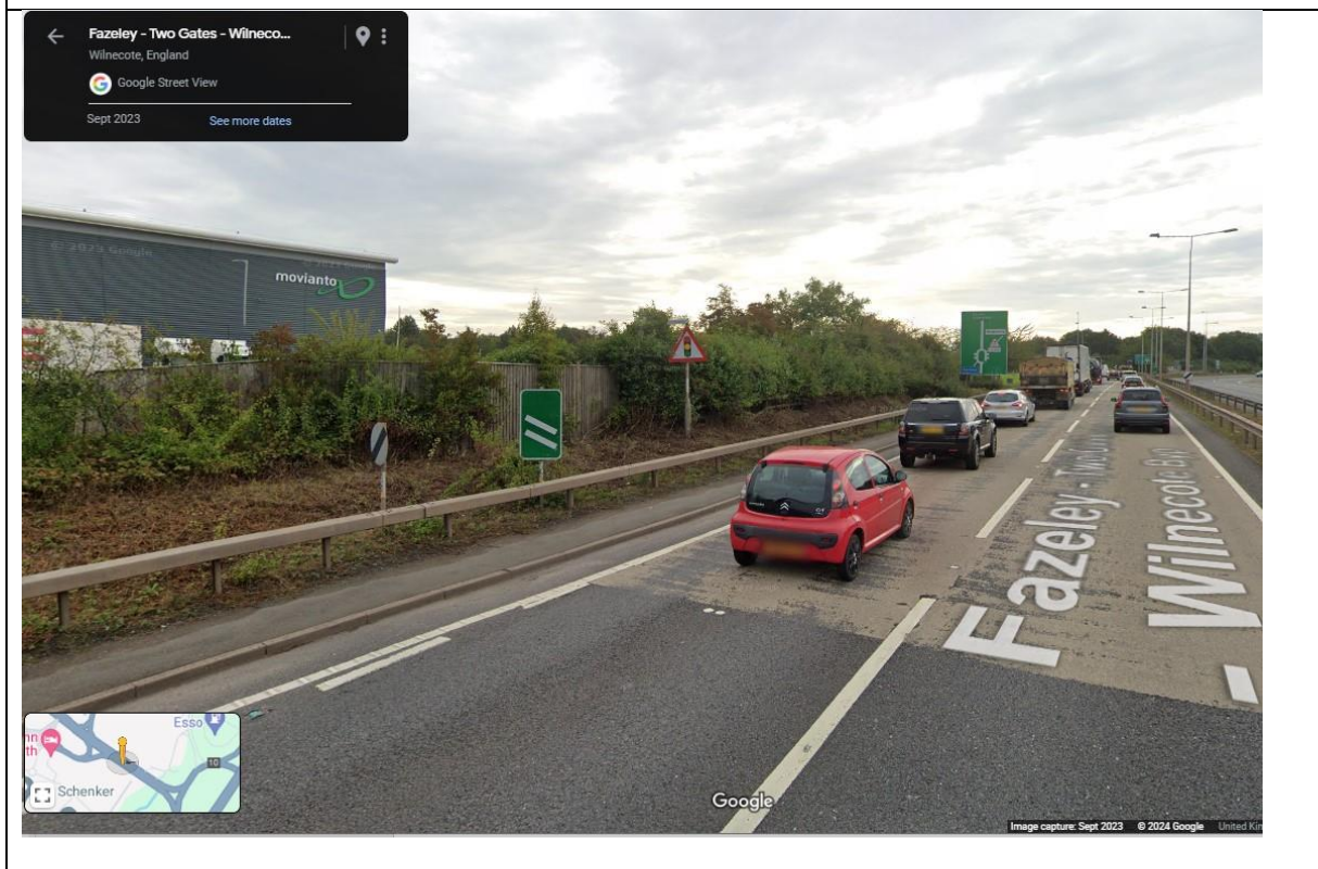
Image 5. Google Street view image of the area of the proposed departures on the A5 eastbound carriageway.
