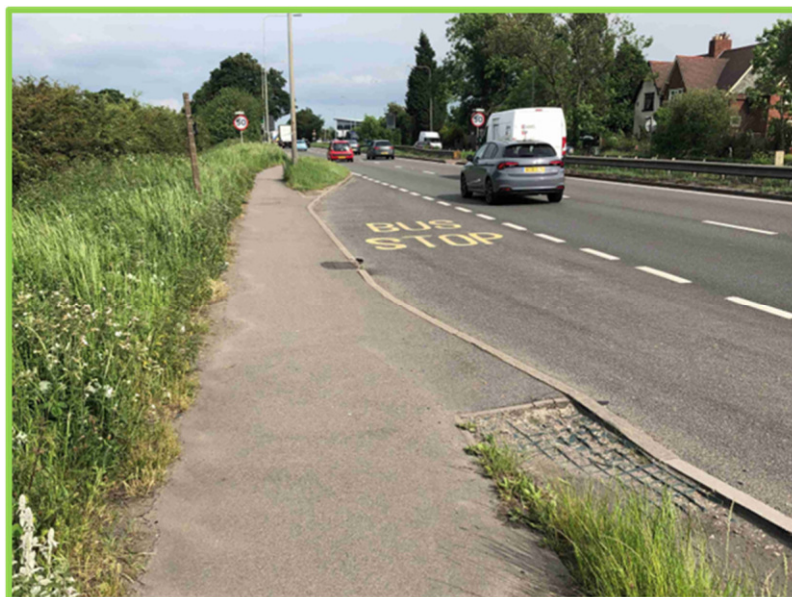
Existing bus stop facilities at A5 eastbound
