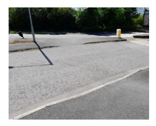
Figure 15 – Absence of tactile paving
