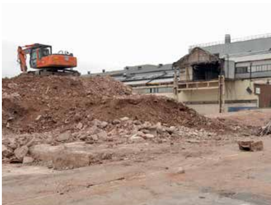
Demolition at Longbridge
