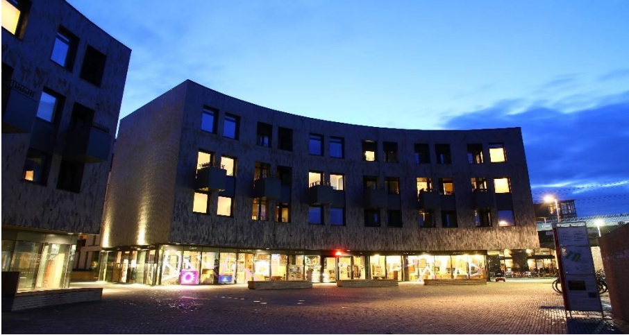
Figure 7.2 City Gate West
