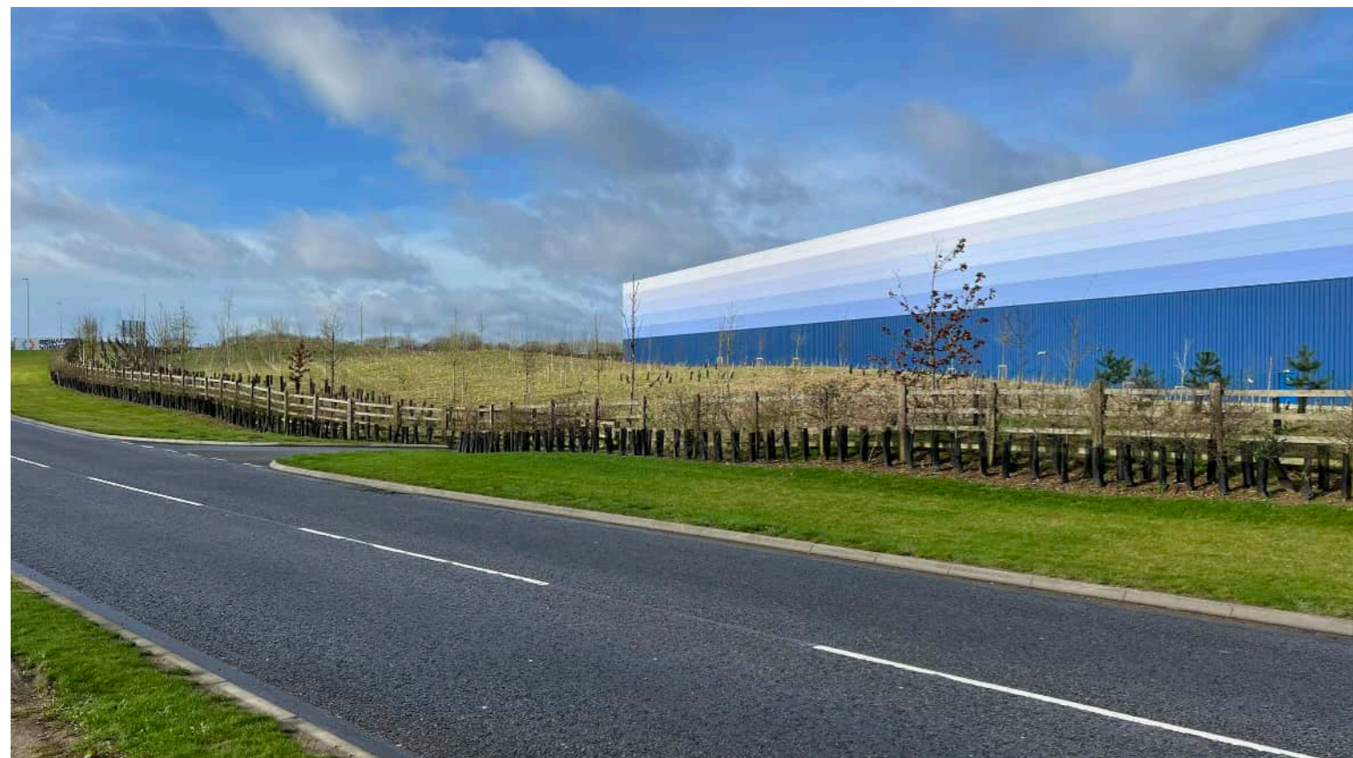
NEW BUNDS AND PLANTING AROUND MAGNA PARK.
