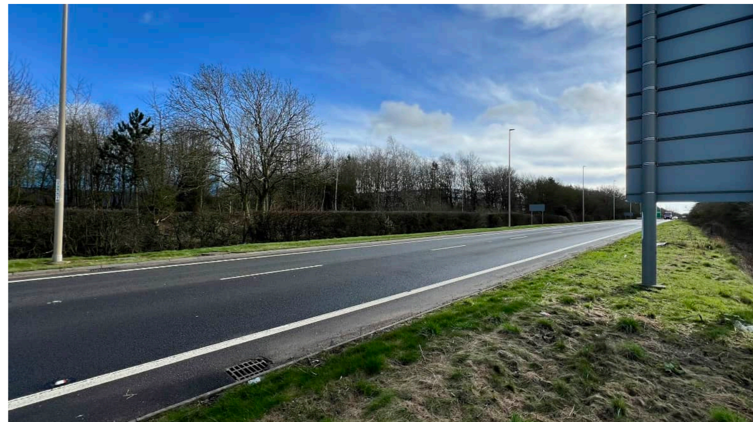
EXISTING ESTABLISHED PLANTING ADJACENT TO THE A5 WITH GLIMPSED VIEWS TOWARDS MAGNA PARK.
