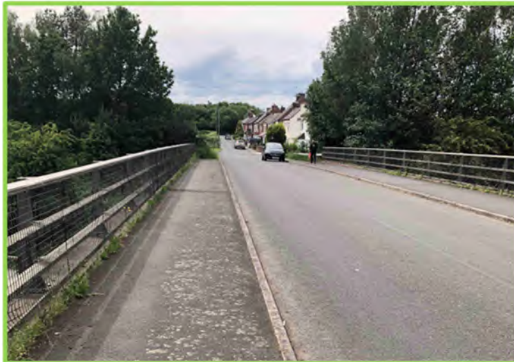
Footways on Green Lane (bridge over M42 motorway)
