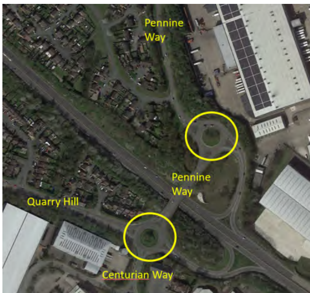
Image 1.1 – Pennine Way Roundabout Junctions
