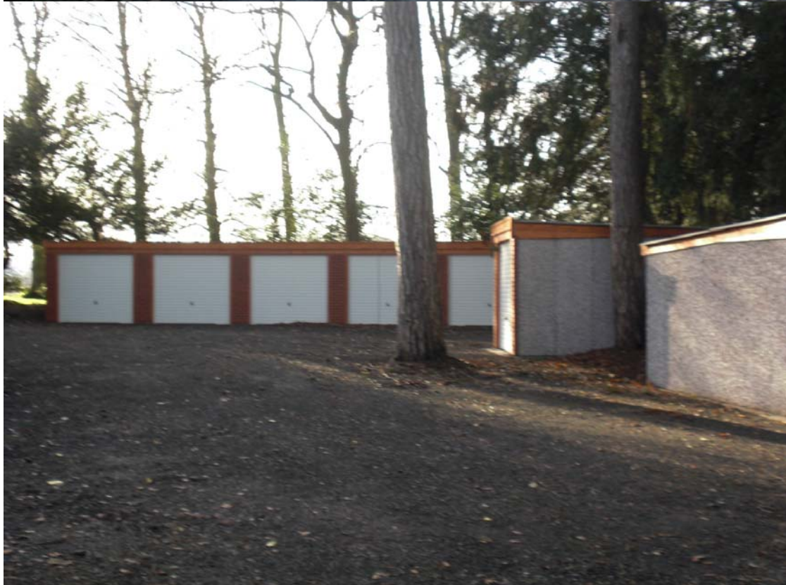
Photos of the garages as built.
