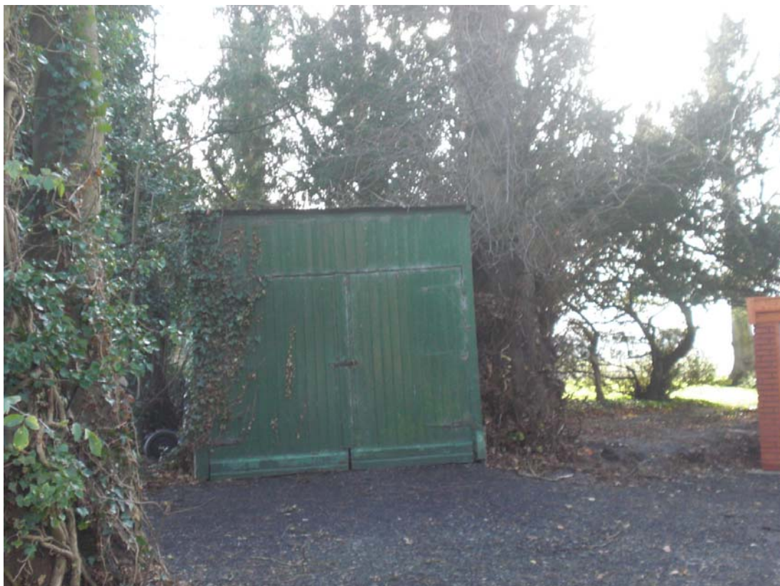
Photo of existing garage that has been retained
