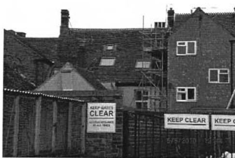
EXAMPLE OF INAPPROPRIATELY LARGE ROOFLIGHTS (REAR OF LONG STREET)
