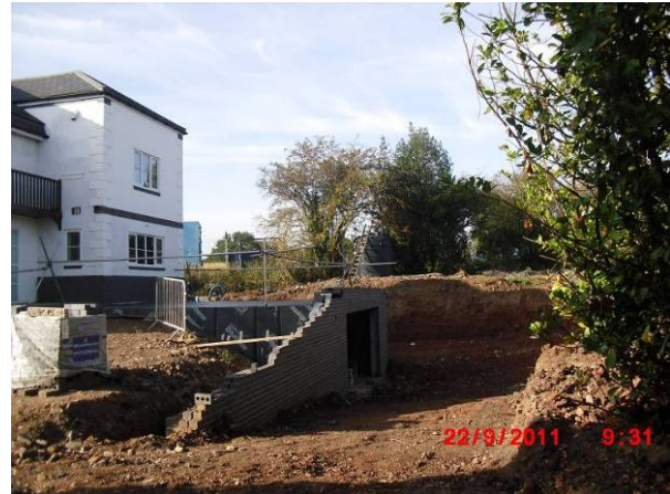
Basement Garage and swimming pool under construction in September 2011
