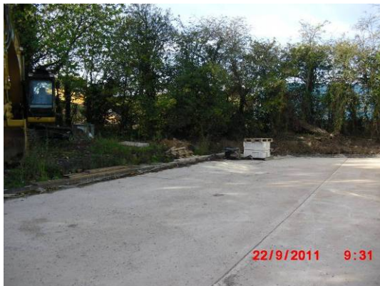
Photograph showing part of the rear surfaced yard.
