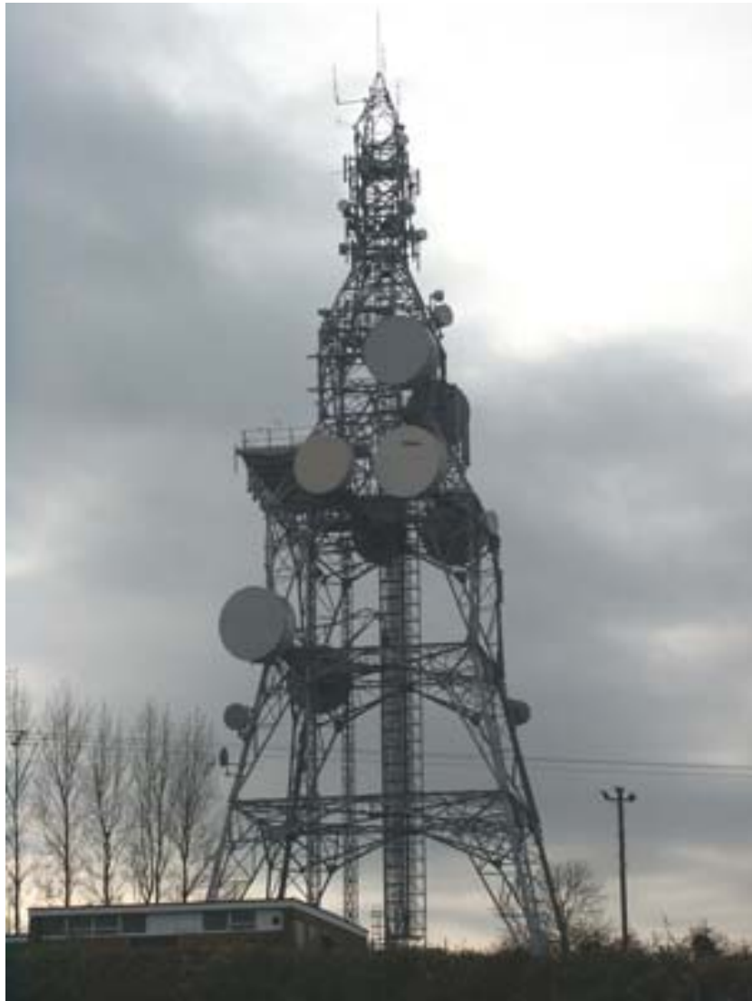
Austrey Microwave Relay Station, north-west of the proposed site
