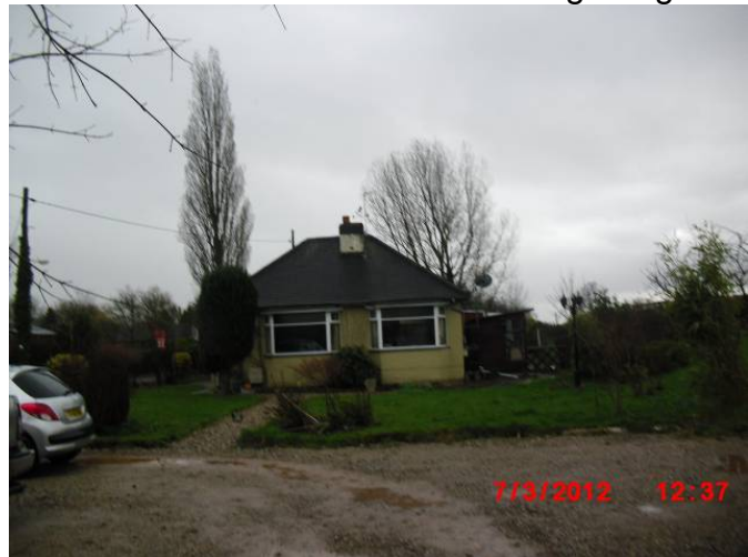
Front elevation of the existing bungalow
