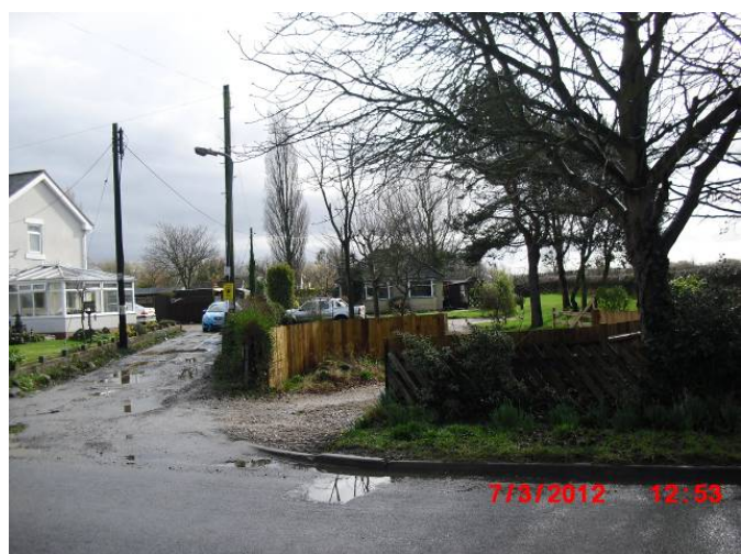
View of existing bungalow showing neighbours dwelling and side road, looking from Birmingham Road
