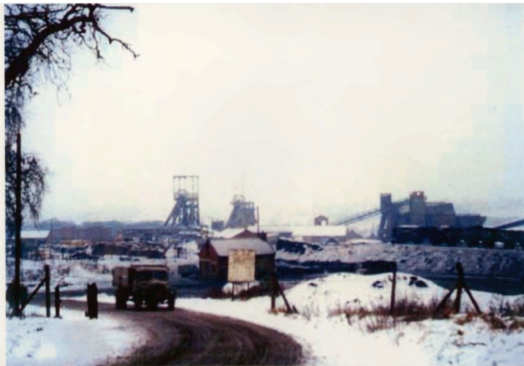
Arley Pit, from Frederick Road January 1963
