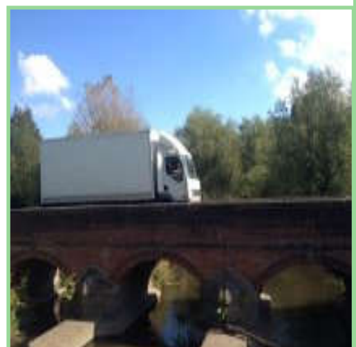
Articulated lorries, trucks and vans over 7.5 tonnes use Coleshill's ancient bridge illegally to access the industrial estate
