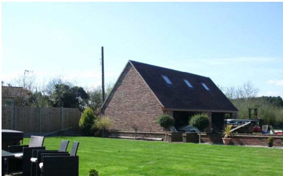
Garage building in-situ
