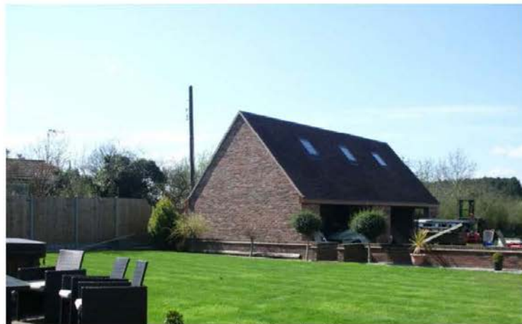
Garage building in-situ
