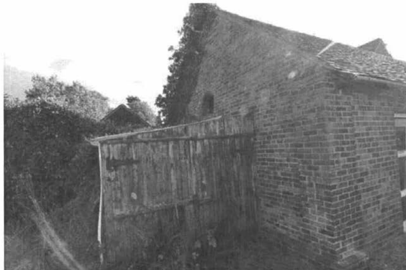
Pl.7: The east gable of the Cart Shed.
