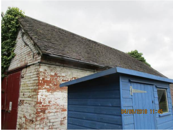
Existing building at site
