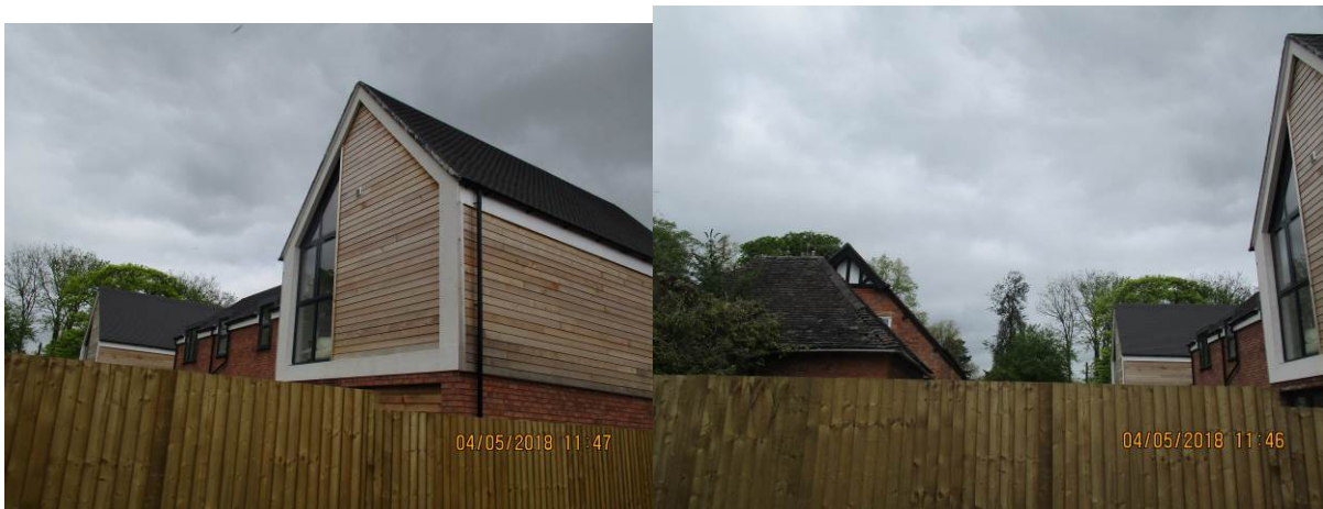
Fence boundary between No. 5 and proposed Plot 2 rear of No. 5 and garden.
