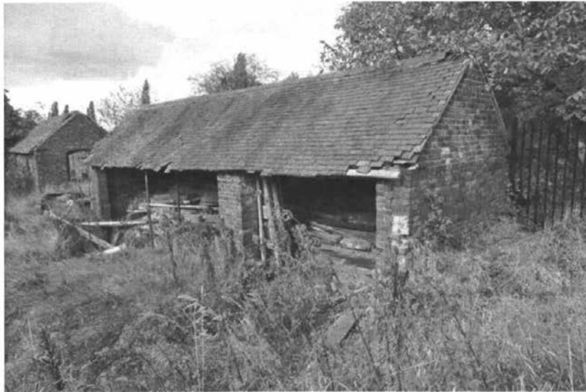
Pl.14: The East Shelter Shed (Building E) from the south-west.
