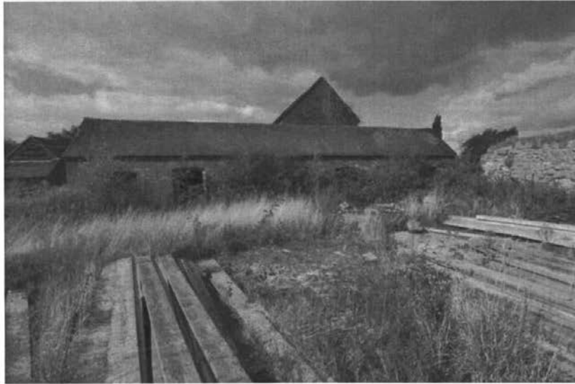
Pl.11: The front, or south, elevation of the South Byre (Building D).
