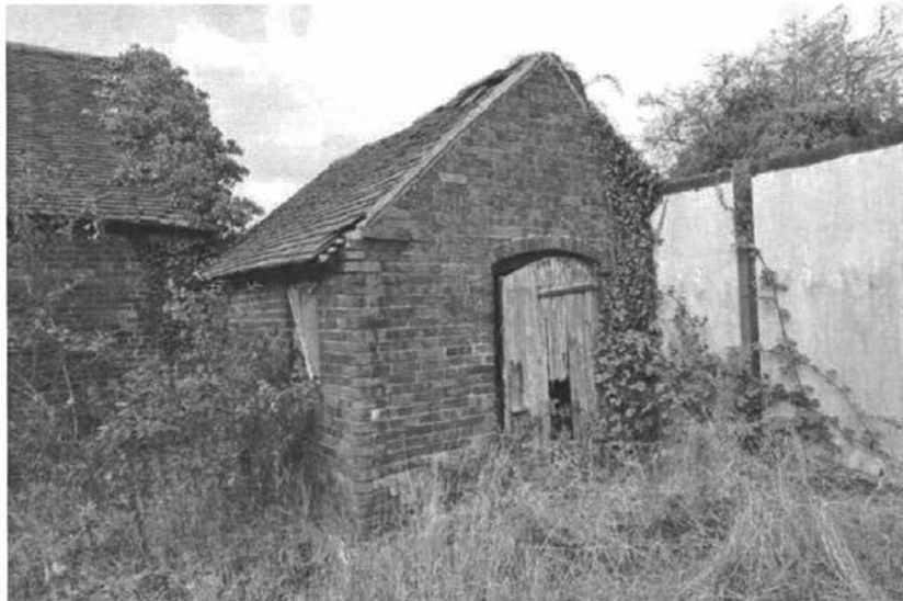
Pl.15: The Loose Box (Building F) from the south-west.
