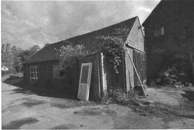
Pl.6: The former Cart Shed (Building B) from the north-west.
