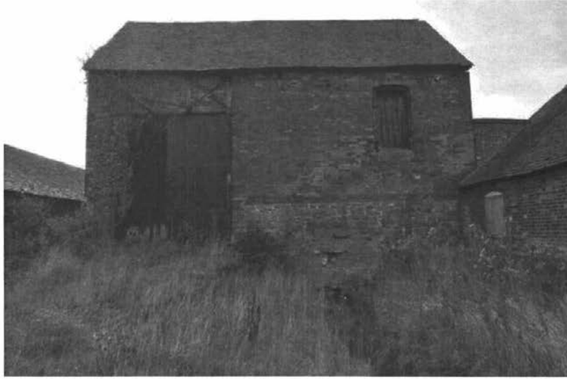
Pl.4: The east elevation of the Barn (Building A).
