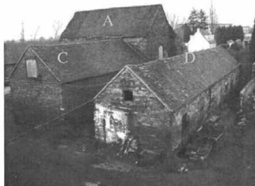
Pl.3: Part of the farmstead to the east of the Hall, forming the north side of the foldyard. The letters relate to the building identification in the report.
