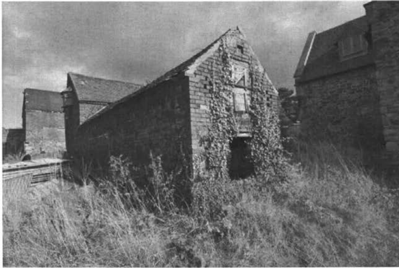
Pl.16: The Piggery complex (Building G) from the north-west, with the main sty range in the foreground; the yards are to the right-hand side.
