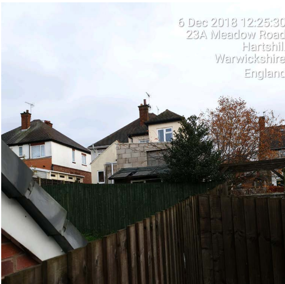
View of structure from Bluebell Close to the rear of the site.
