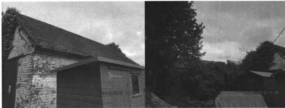
Existing building at site
