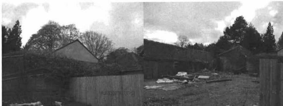
Wall boundary between Mews and Application site
