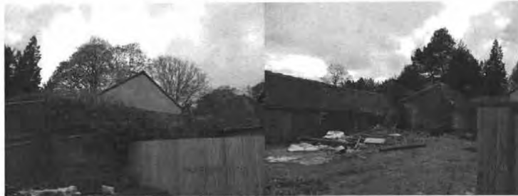
Wall boundary between Mews and Application site
