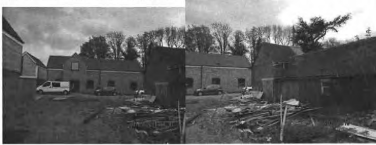
From application site towards No. 1 Hawcutt No.1 Existing building on east side of application site towards No.1
