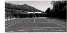
Anti slip acrylic coating to be applied. Colours to be similar to existing.
