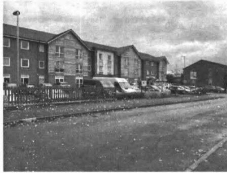
Church Hill opposite the building materials yard and asphalt yard
