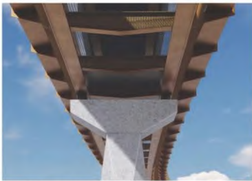
Figure 45: Solid plate over the viaduct piers to direct rainwater away from the concrete
