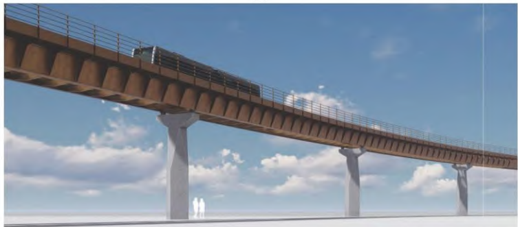
Figure 45: Solid plate over the viaduct piers to direct rainwater away from the concrete
